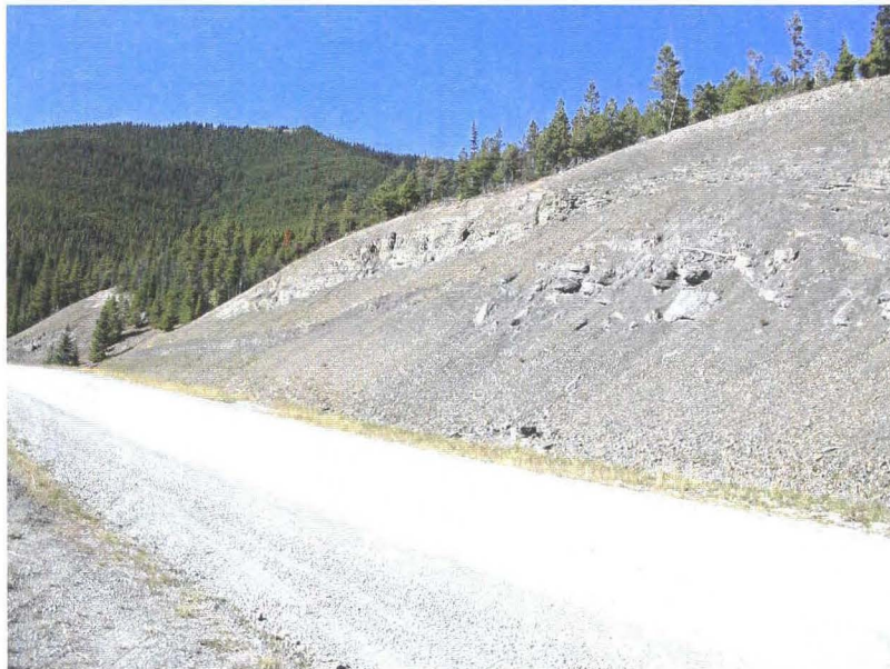
Photo 940-16 (bottom) – Facing southbound across the Km 20.2 Cut Slope site.
