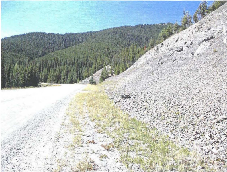
Photo 940-17 (top) – Facing southbound along the ditch at the Km 20.2 Cut Slope site. Note the debris accumulation into the upslope side of the ditch.
