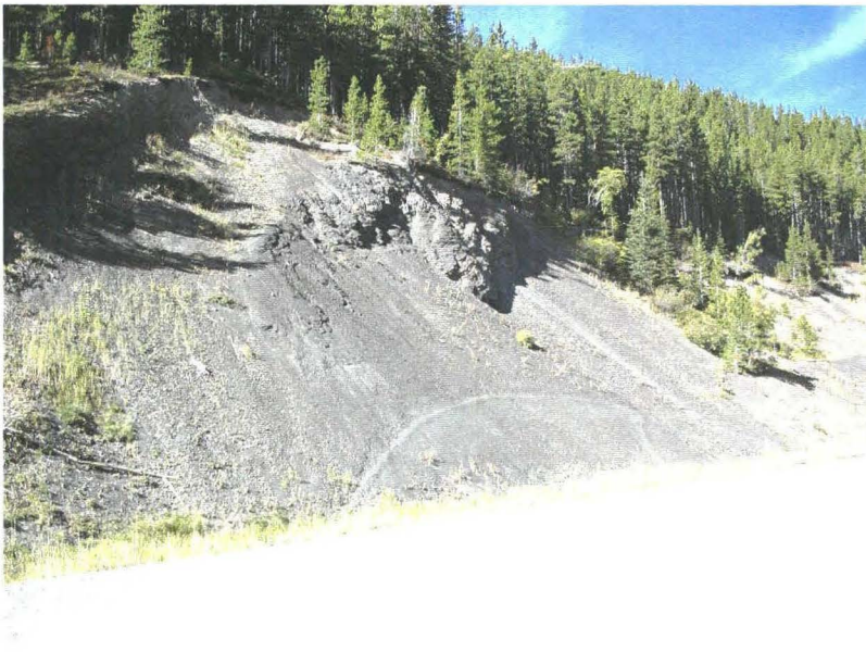
Photo 940-10 (bottom) – Closer view of the Km 15 Cut Slope site. Note the bedrock exposed in the upper portion of the cut slope, and the apron of debris covering the lower portion of the cut slope.
