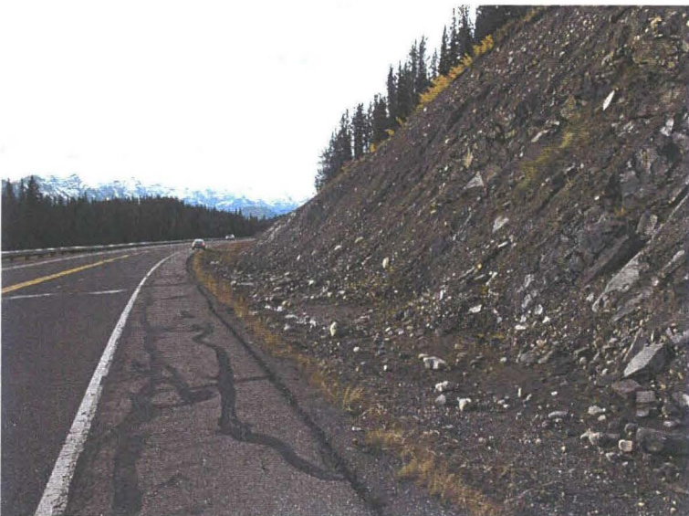
Photo 2 (middle) – Facing northwest across the northern end of the cut slope. Note the proximity of the debris in the ditch to the edge of the pavement.
