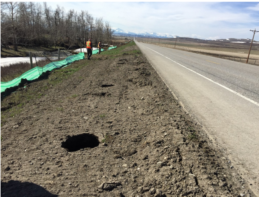
Photo 6 Sink holes up to 1 m deep where noted across all 4 sites due to the recent construction activities. The contractor who installed the sheet piles were contacted instructed to get these remediated as soon as possible.
