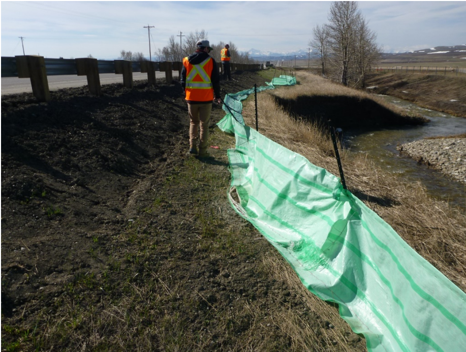
Photo 2 Site C (north) – Erosion has occurred in a side channel which had some ponded water at the time of inspection. Main channel 15 m to right of side channel. Sheet pile wall installed 1.5 m off the highway shoulder. Photo was taken facing north on May 2, 2018.
