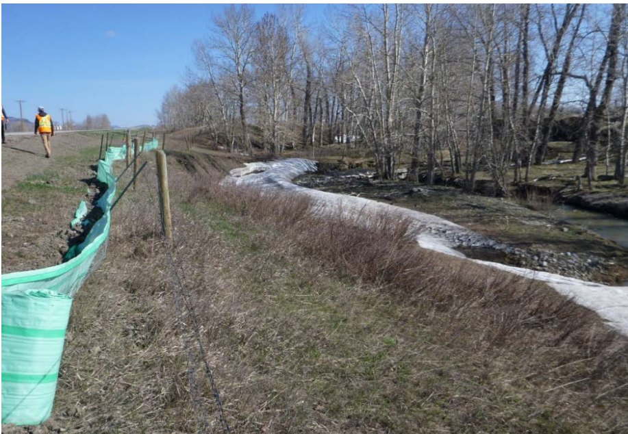
Photo 2 Site C (north) – Erosion has occurred in a side channel which had some ponded water at the time of inspection. Main channel 15 m to right of side channel. Sheet pile wall installed 1.5 m off the highway shoulder. Photo was taken facing north on May 2, 2018.
