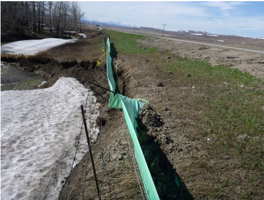
Photo 4 Site B - erosion scarp undermining fence with retrogressing back scarp instability approaching ditch. Sheet pile wall installed 1.5 m off the highway shoulder. Photo was taken facing north west on south on May 2, 2018.
