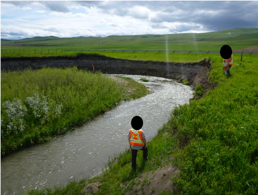
Photo 5 Site A - erosion scarp undermining fence with retrogressing back scarp instability extending into ditch. Note orange-cased utility cable undermined by erosion. Photo was taken facing north east on June 1, 2017.
