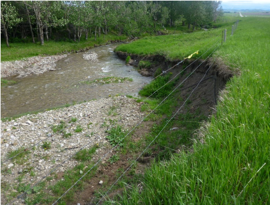
Photo 4 Site B - erosion scarp undermining fence with retrogressing back scarp instability approaching ditch. Photo was taken facing north west on June 1, 2017.
