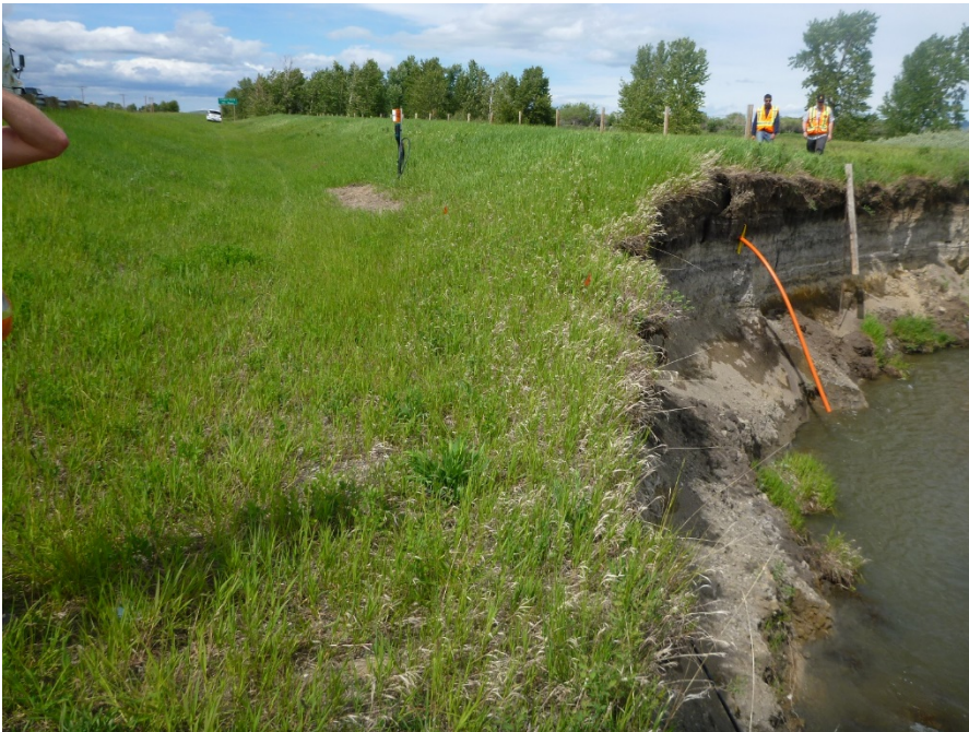
Photo 5 Site A - erosion scarp undermining fence with retrogressing back scarp instability extending into ditch. Note orange-cased utility cable undermined by erosion. Photo was taken facing north east on June 1, 2017.
