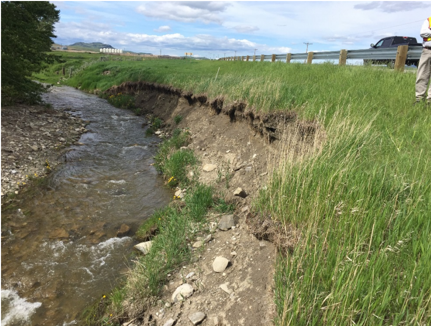
Photo 2 Site C (north) – Erosion has occurred in a side channel which had some ponded water at the time of inspection. Main channel 15 m to right of side channel. Gravel bed and scour hole formed and erodible material in cut bank. Photo was taken facing south on June 1, 2017.
