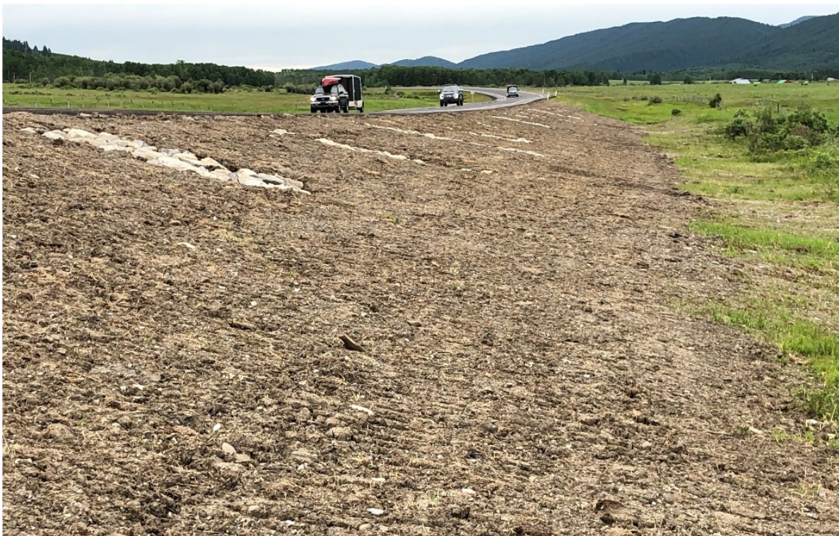
Photo 2 West slope has been stripped and regraded as part of ongoing highway overlay project. Photo taken facing south along the west side on July 7, 2020.
