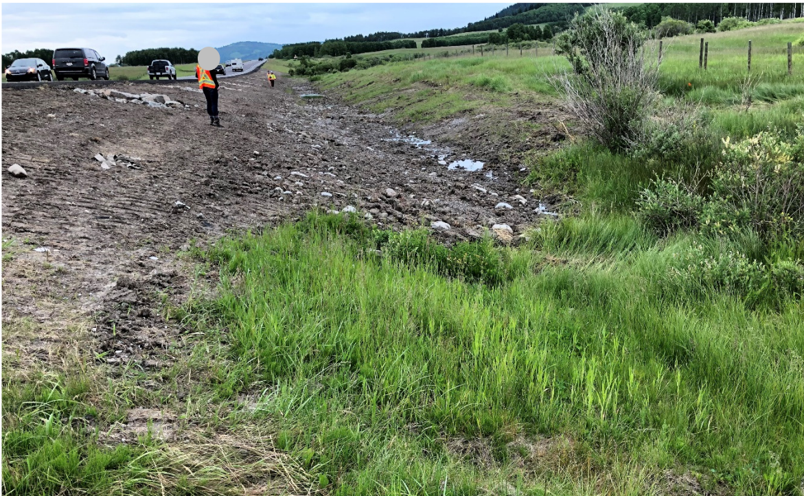
Photo 4 Seepage and saturated ground on the east slope. Standing water in the ditch due to poor grading of the ditch. Photo taken facing north on July 7, 2020.
