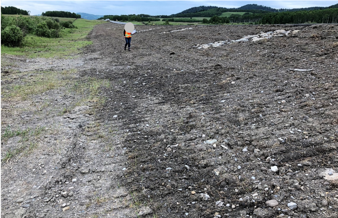
Photo 4 Seepage and saturated ground on the east slope. Standing water in the ditch due to poor grading of the ditch. Photo taken facing north on July 7, 2020.
