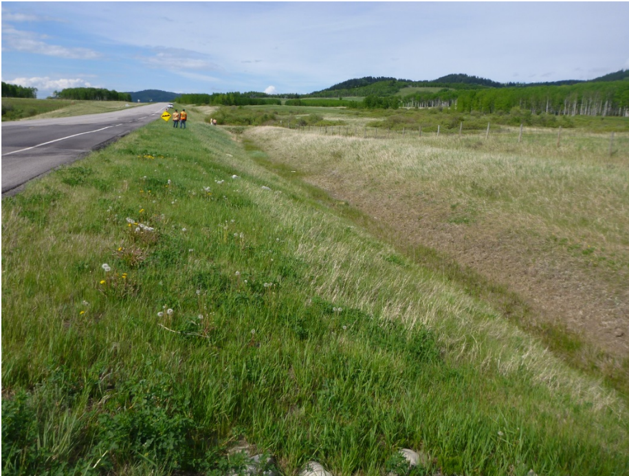
Photo 4 Base of ditch on east side of highway. Ditch unable to drain due change in ditch grade before culvert. Photo taken facing north on June 1, 2017.
