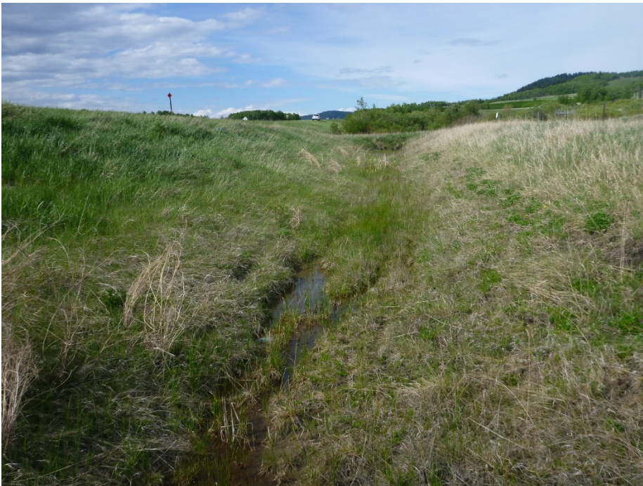
Photo 4 Base of ditch on east side of highway. Ditch unable to drain due change in ditch grade before culvert. Photo taken facing north on June 1, 2017.
