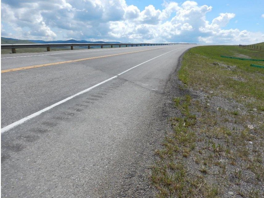
Photo S38-3 (May 2015) – Facing south from the west side of the highway. New pavement overlay placed in 2014 was in good condition.
