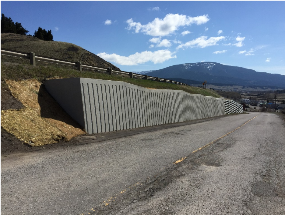
Photo 2 Voids behind the previous steel wall have been filled in. The photo was taken facing southeast on May 2, 2018.
