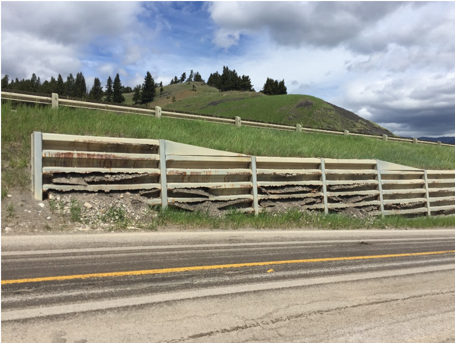
Photo 2 East extent of bin wall. Moving from west to east, the corrosion severity decreases. The photo was taken facing northeast on June 1, 2017.
