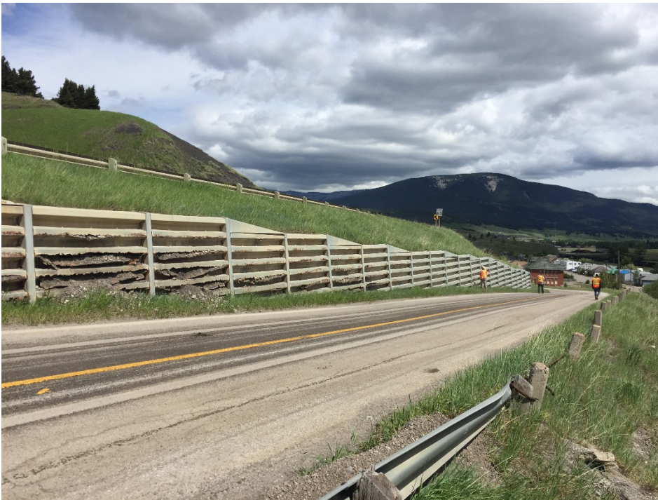
Photo 2 East extent of bin wall. Moving from west to east, the corrosion severity decreases. The photo was taken facing northeast on June 1, 2017.
