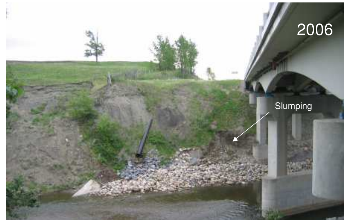
Photo S1-4 – June 2006 (lower right) East creek bank, as seen during the 2006 inspection.
