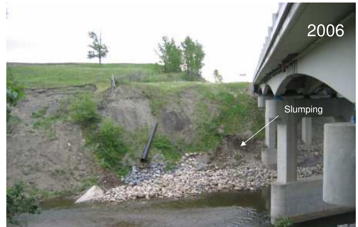
Photo S1-4 – June 2006 (lower right) East creek bank, as seen during the 2006 inspection.
