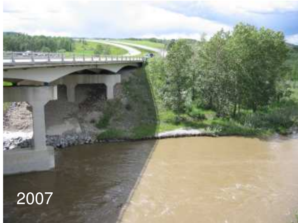
Photo S1-1 – June 2007 (upper left) West creek bank, downstream of the westbound bridge. Note the erosion visible along the unarmoured segment of the creek bank in comparison to the 2005 photo of the same area (Photo S1-2).
