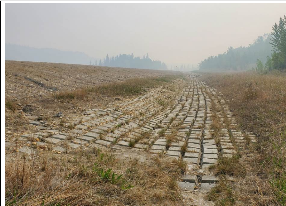
Photo 7-15. Looking east towards cabled concrete section (32+700). Section was performing well. Minor erosion damage was noted on the north side of the ditch. No major change from the 2020 condition.
