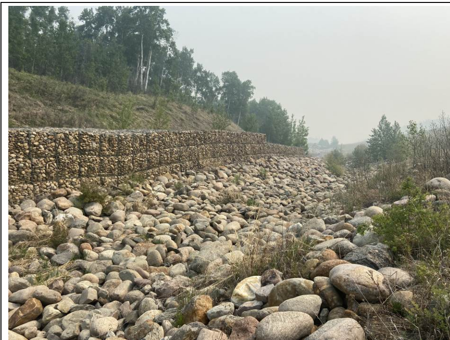
Photo 7-01. Gabion retaining wall and armoured channel observed in good condition (32+310).
