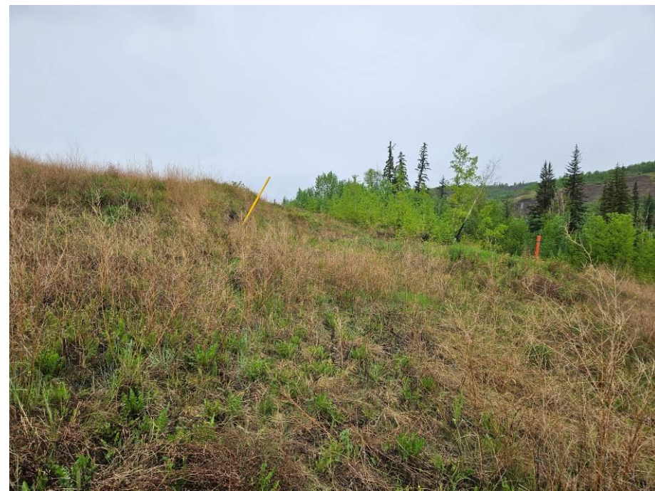
Photo 43-02. Main slide scarp of active shallow failure downslope of the buried pile wall (33+325) first observed in 2017. Area is vegetated but appears there is active movement within the disturbed slide mass. No scarp retrogression since 2023.
