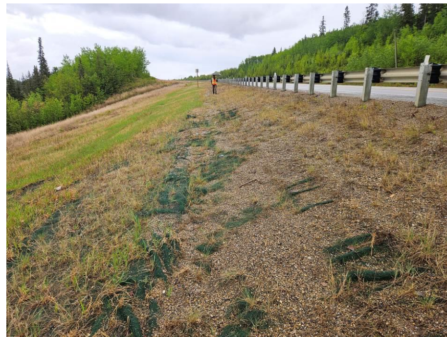
Photo 43-14. Looking east towards the TRM installation on the upper portion of the slope north of the road (33+800). Limited vegetation growth within the upper road embankment likely due to sand and salt runoff from winter road maintenance.
