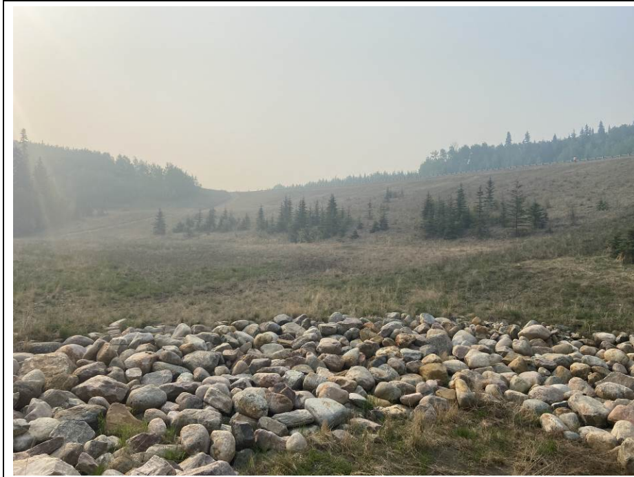
Photo 43-07. Looking south towards the Site B highway embankment and overland flow area. Minor rill erosion is visible on the right top corner of the photo along the slope.
