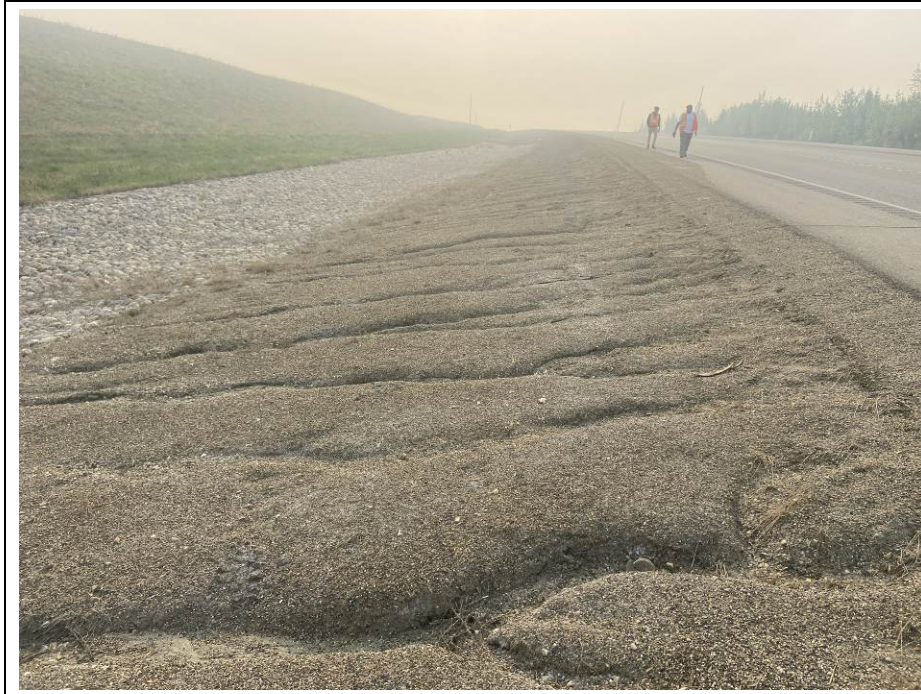
Photo 43-19. Rill erosion between the road and north ditch gabion armour (km 34+000) was slightly worse compared to the 2022 condition. TRM should be added to reduce rates of erosion.
