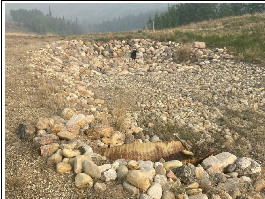
Photo 43-11. View of culvert inlet and riprap protection near 33+900 on north side of road.
