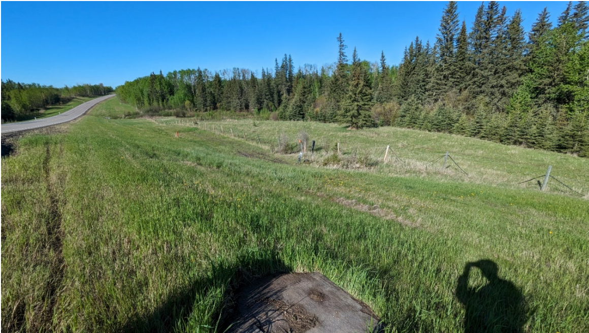
Photo 5 – Looking southwest downslope of the highway surface.
