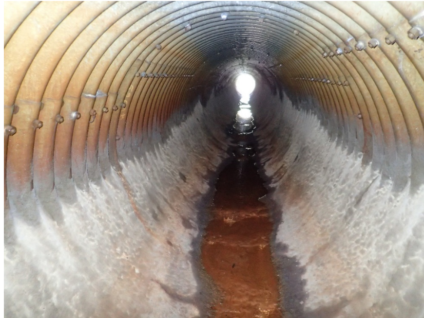
Photo 7: Walk through of culvert conducted and indicated no obvious sidewall distortion.
