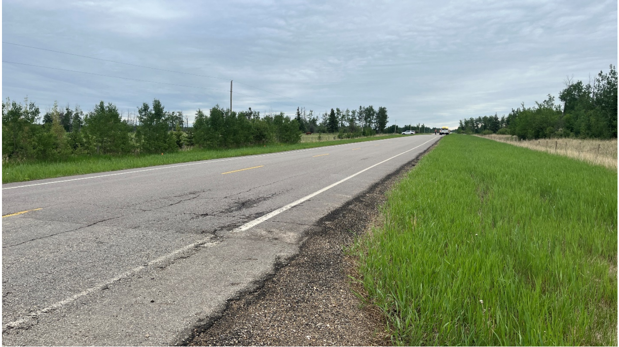
Photo 1 – Looking southeast along SBL at the north end of the site.
