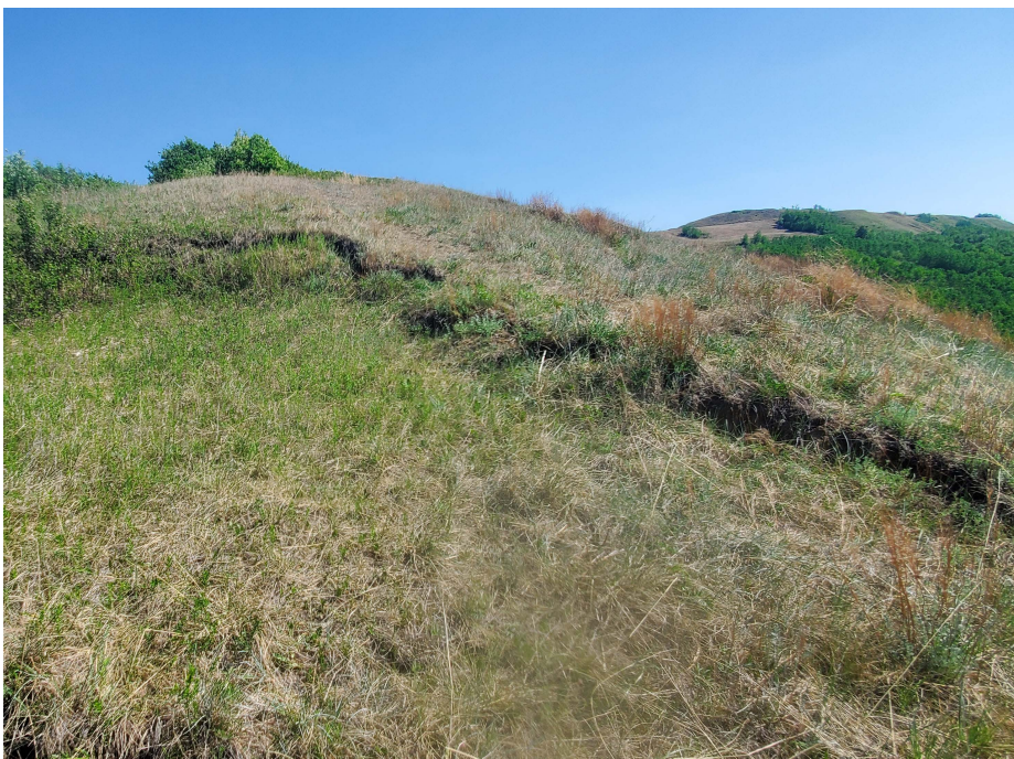
Photo 7. Looking east at one of three tension cracks observed upslope from the slide scarp in previous photo. The crack was opened up to 0.4 m wide and with up to 0.3 m of drop. Will likely become the main head scarp in the future.
