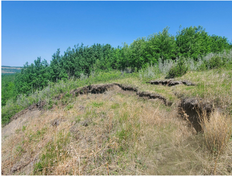
Photo 6. Slide area (first observed in 2019) approximately 100 m NW of the north end of the pile wall. No major change at the main scarp since the 2021 inspection; ongoing creep movement further downslope.
