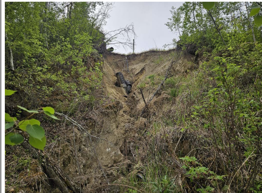
Photo 5. Looking southwest from below the scour gully headwall caused by the breakage in the CNR CPP Trunk pipe. There has been some retrogression and lateral expansion at the gully headwall since 2023.
