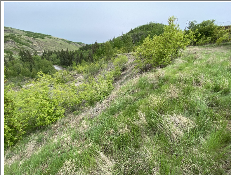
Photo 6. Looking southeast from the north side of the lower slide main scarp. No major changes observed in the slope area directly below the pile wall since 2023.
