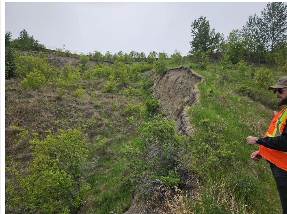
Photo 9. Looking west at the slide lower slide mass. There was some increased erosion along the slide flank relative to the 2023 condition but no major expansion.
