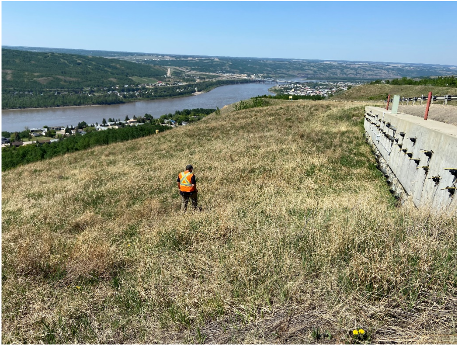
Photo 9. Looking north at the bench and graded area below the “Makeout” pile wall. Area appeared in good condition and had no observable changes from 2021.
