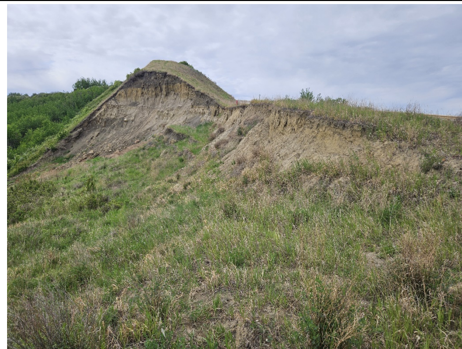
Photo 4. Looking south along the landslide backscarp at the top of the Heart River valley on Hwy 744:04 at km 57.85. There was a slightly larger buildup of soil at the base of the vertical scarp, indicative of ongoing erosion but no major lateral expansion or retrogression towards the highway since 2023.
