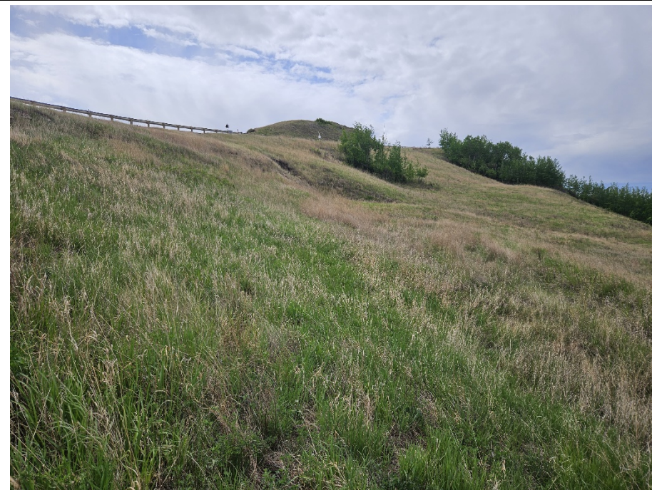
Photo 8. Looking south near km 57.8 along the west side slope of the below the highway with active gully erosion and old, vegetated slide scarps. No major visible difference in the slide terrain within the upper slope relative to the 2023 condition.
