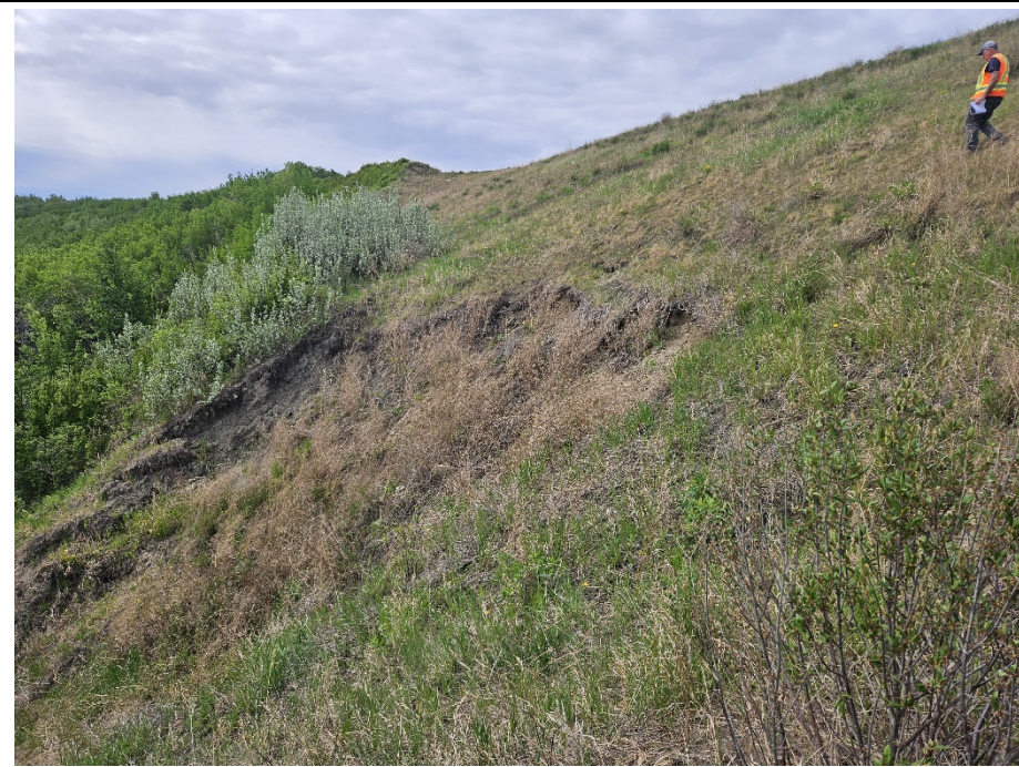
Photo 12-07. Looking south at earth flow at Main Slide 3. No significant retrogression or expansion of the main scarp since 2023.
