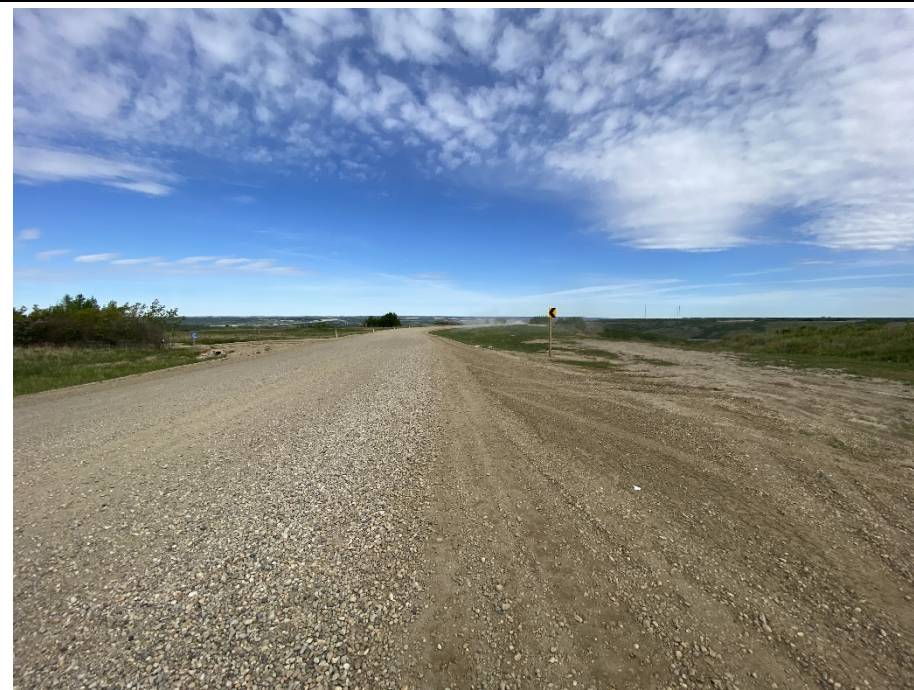
Photo 12-09. Standing within the gravel realignment looking north from the south end of the site. Barriers or a guardrail should be considered at the road bend here (KM 56+000 to 57+000) for northbound traffic to reduce potential for drivers to maintain a course into the old alignment.
