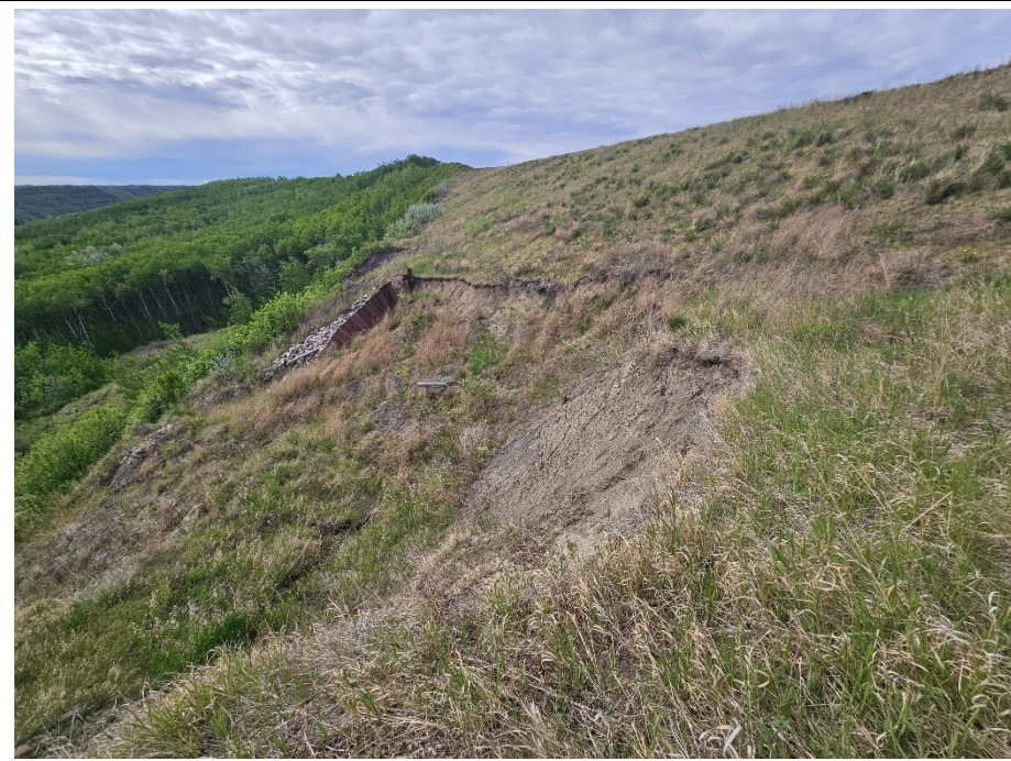
Photo 12-04. Looking south at Main Slide 2 and 2.1 from the north end of Heart River Landslide repair excavation (Former Slide 2). Ongoing downslope movement and minor scarp erosion but no major retrogression / expansion of the scarp relative to the 2023 condition.
