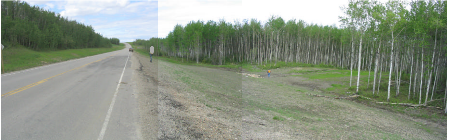
PHOTO 1 LOOKING NORTH TO NORTHEAST AT RECENTLY REPAIRED SITE
