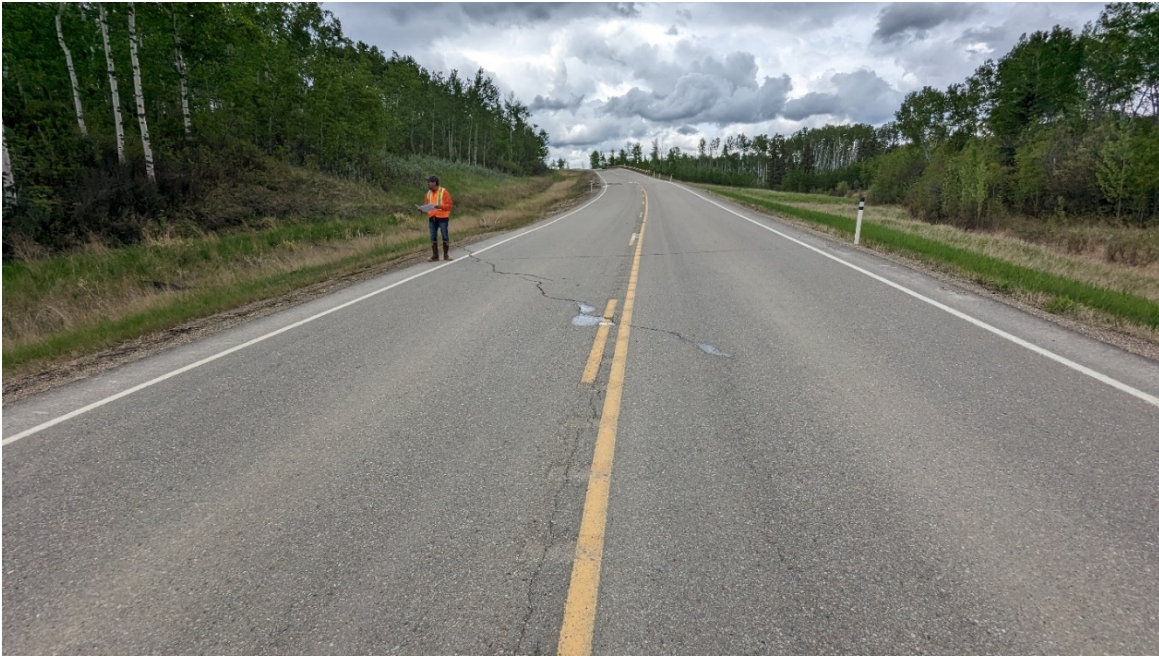
Photo 1 – Looking northeast from the southwest end of Site 11.
