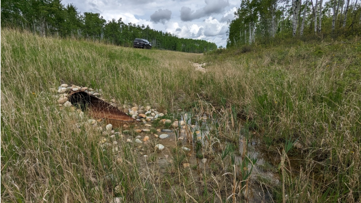
Photo 1 – Looking northeast along downslope ditch.
