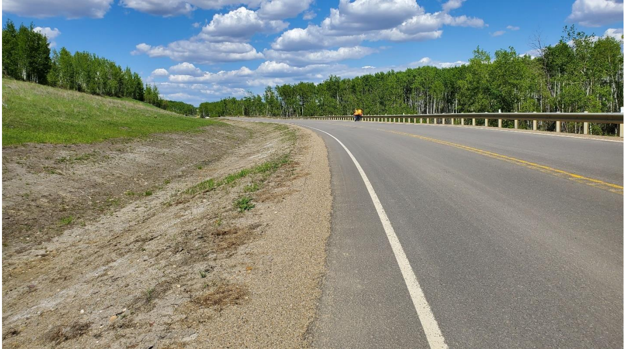
Photo 3 – Looking up-chainage where overlay has covered previously-observed cracks.
