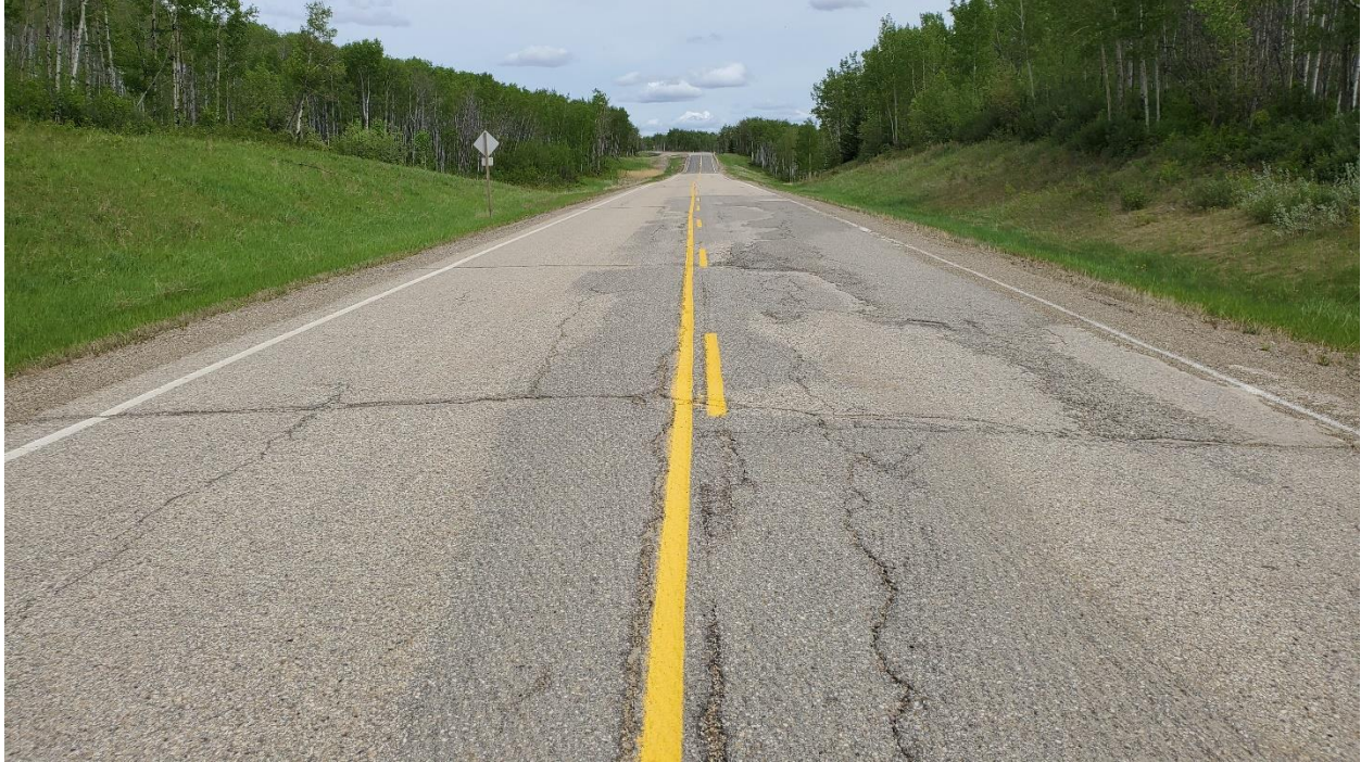
Photo 5, Site 5 – Looking northeast at partially-milled patch between km 19.10 to km 19.13.
