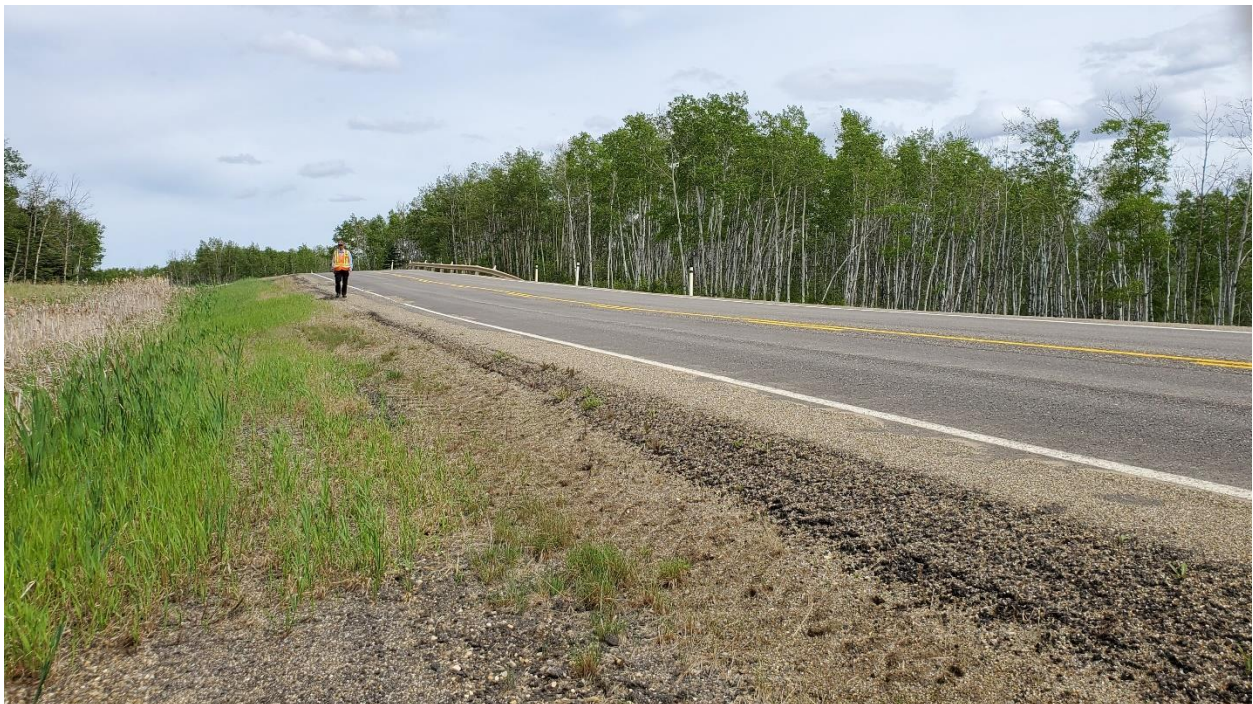
Photo 10, Site 6 – Looking east at 2019 patch near east end of site.
