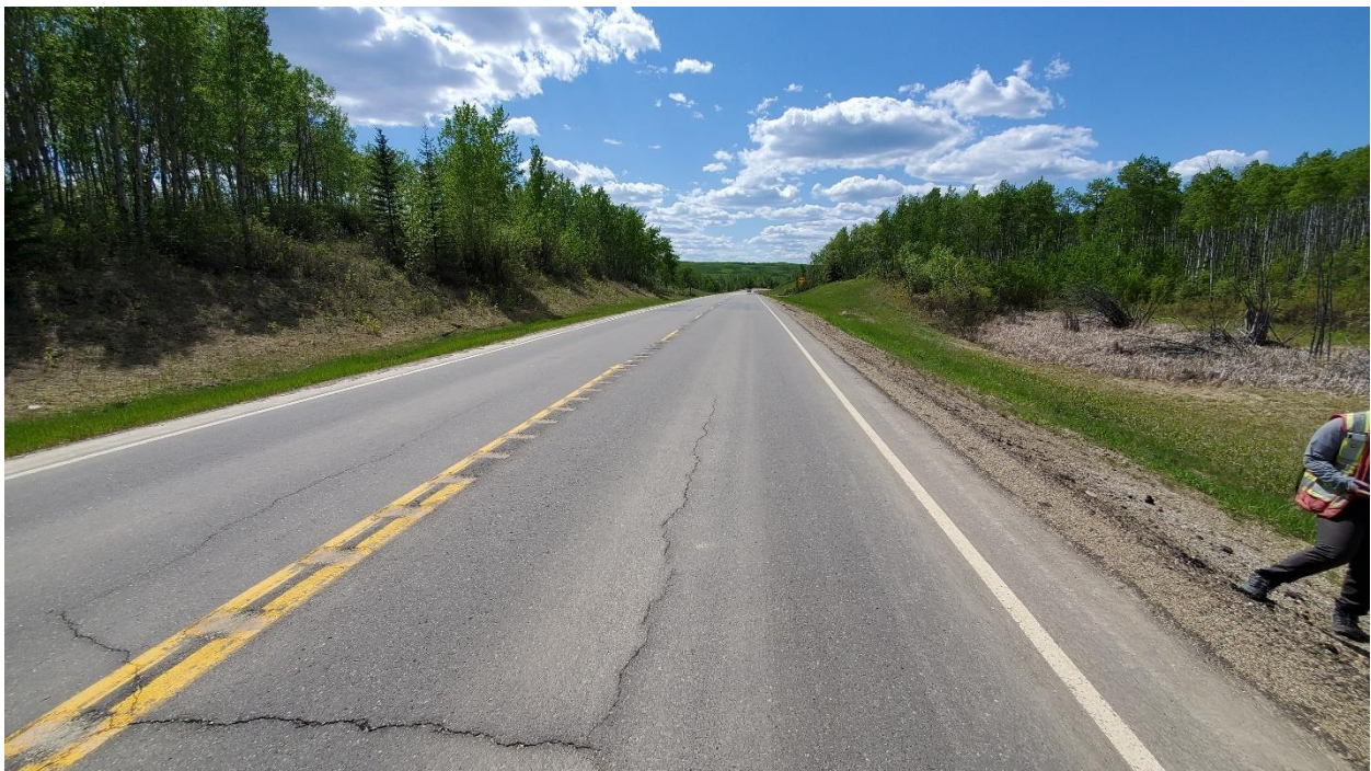
Photo 8, Site 6 – Looking west at west end of Site #6 toward Site #5.
