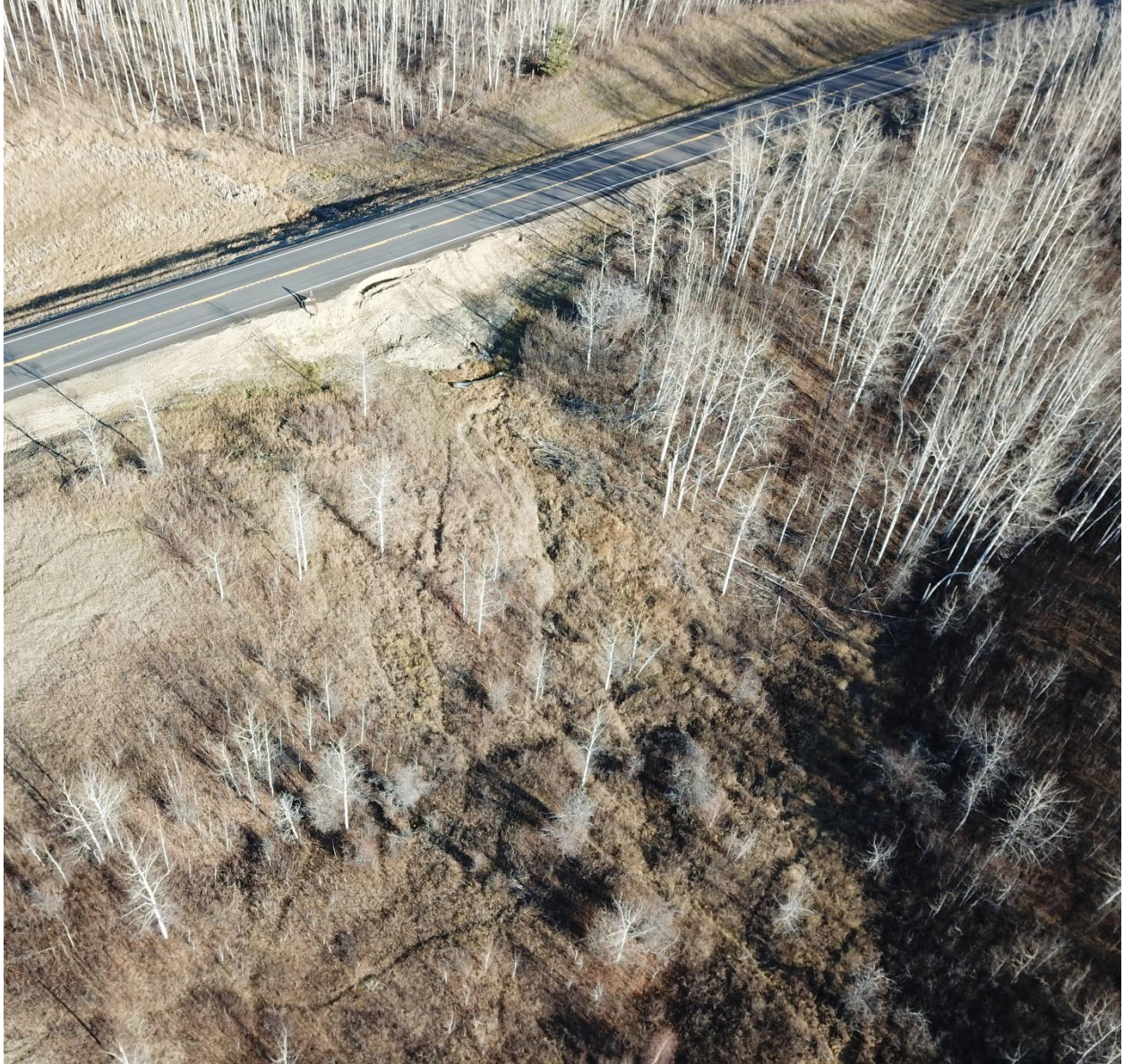
October 28, 2021 - UAV Oblique Photo of slump, gully, and sag pond.
