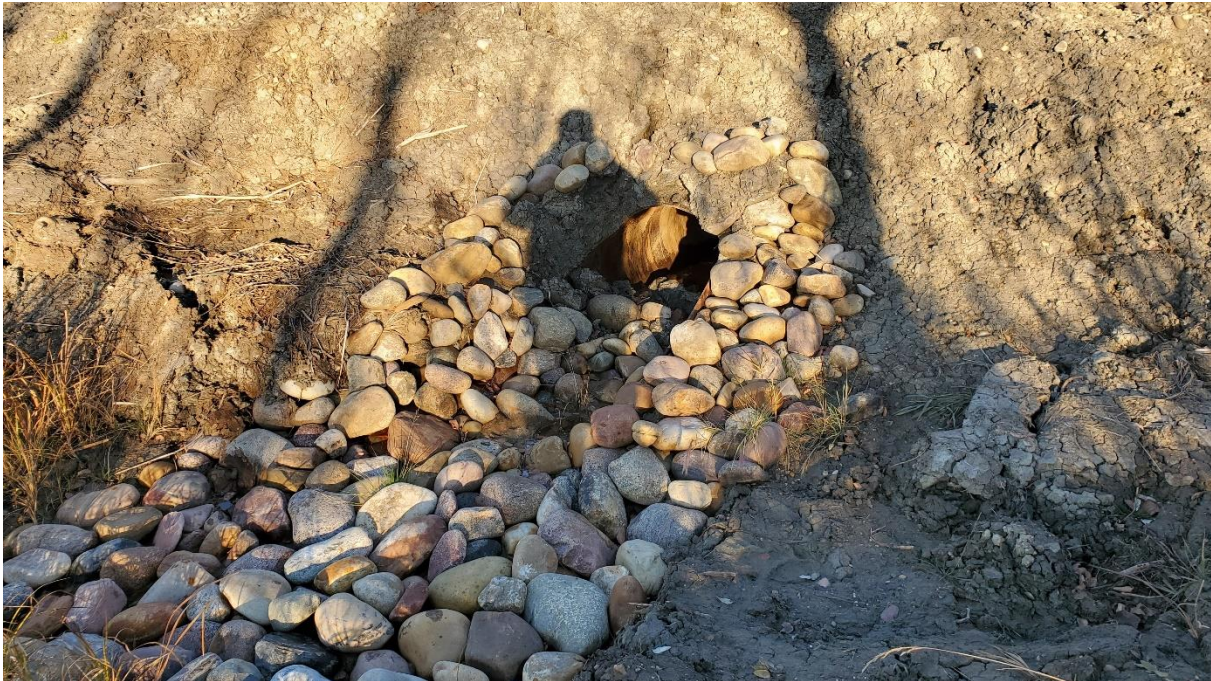
Photo 5 (Oct. 28) – Toe roll around culvert outlet
