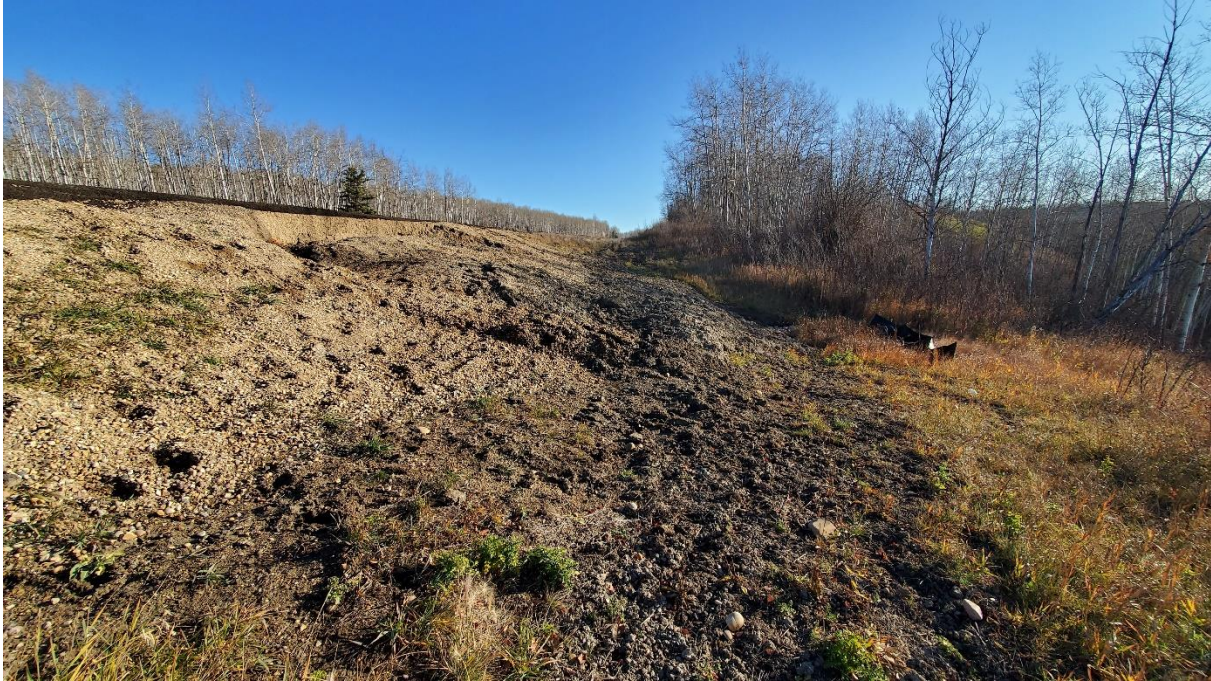
Photo 7 (Oct. 28) – Looking west at profile of the slide.
