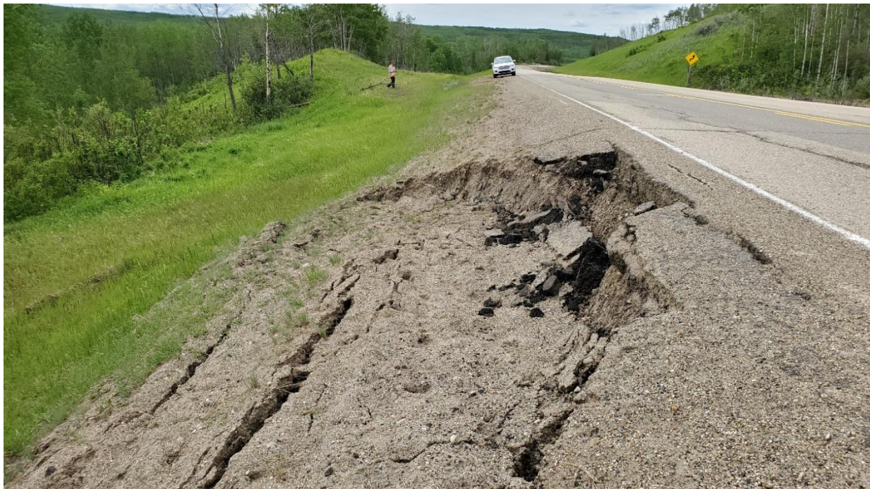
Photo 4, Site 5: Looking west at new slide over the culvert outlet at km 19.07.
