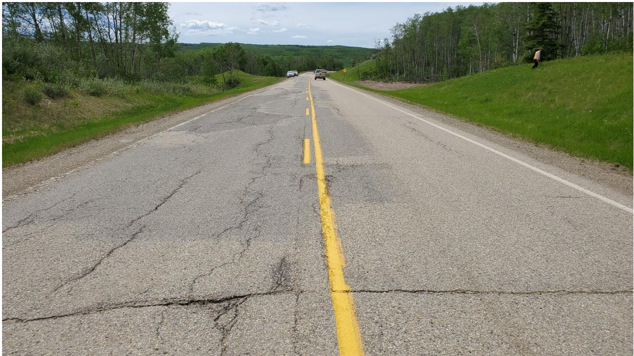
Photo 6, Site 5 – Looking southwest at milled patch between km 19.10 to km 19.13.
