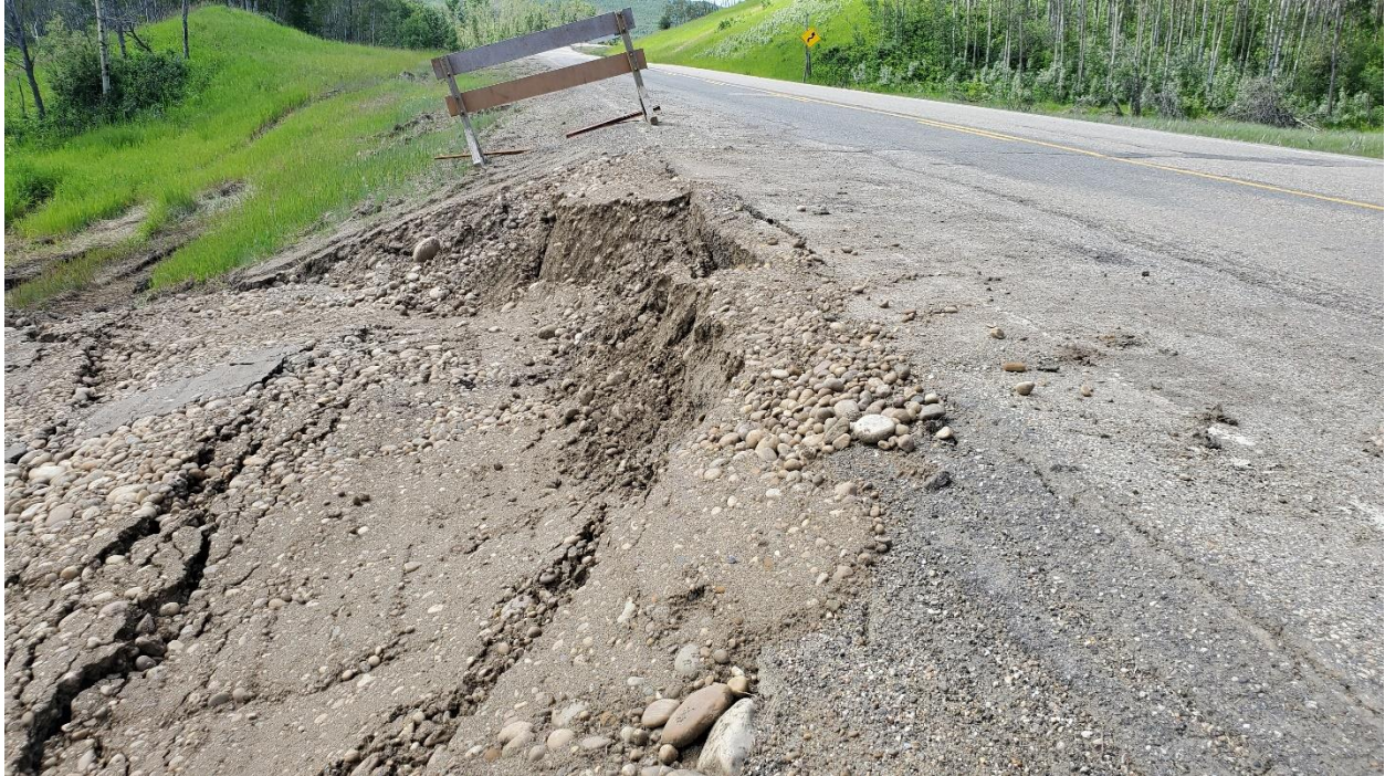
Photo 4, Site 5 (June 24, 2020): Looking west after emergency fill placement.
