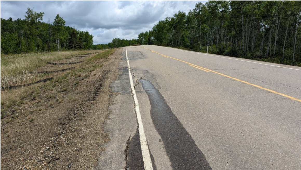
Photo 7, Site 6 – Looking northeast at matting and GeoRidges installed in the north ditch. Cracking observed through patches along the fog line.
