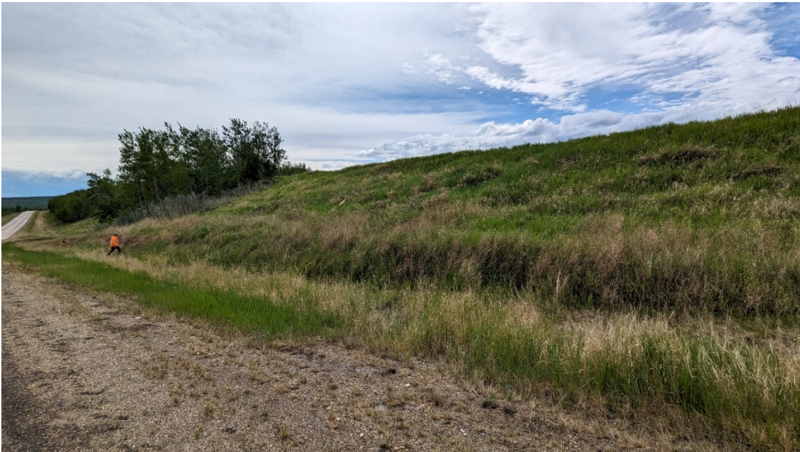
Photo 8, Site 15 – Looking southwest at backslope slump at valley crest.
