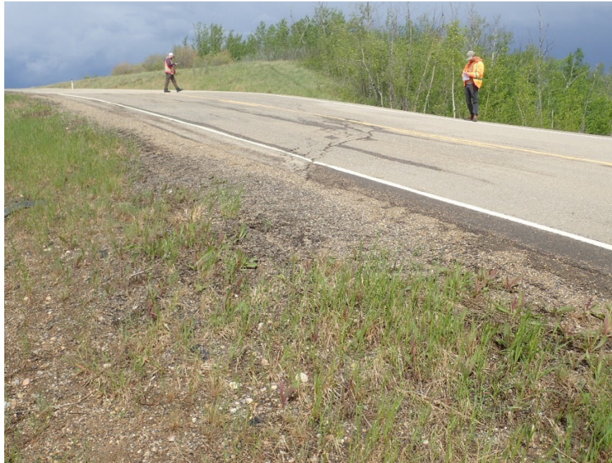
Photo 7, Site 15 – Looking northeast where scarp from road extends southwest into the treeline
