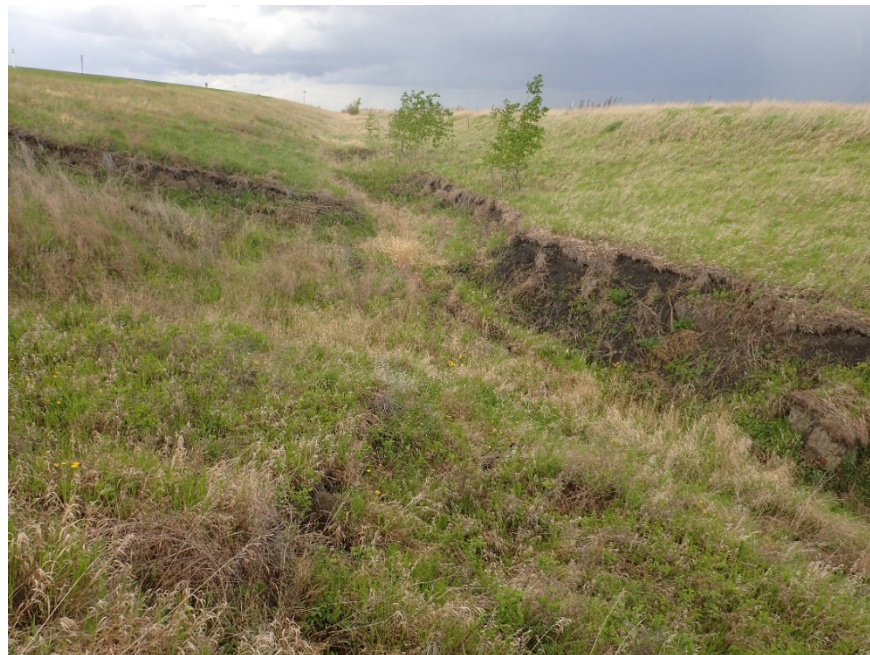
Photo 2, Site 14 – Looking north along the east ditch.
