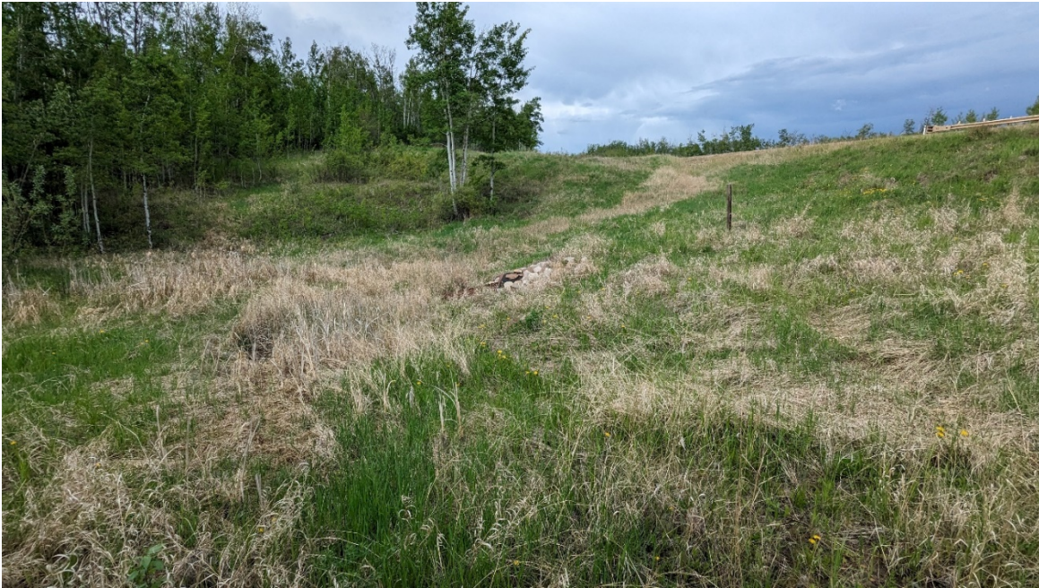
Photo 3: Looking north at culvert inlet.
