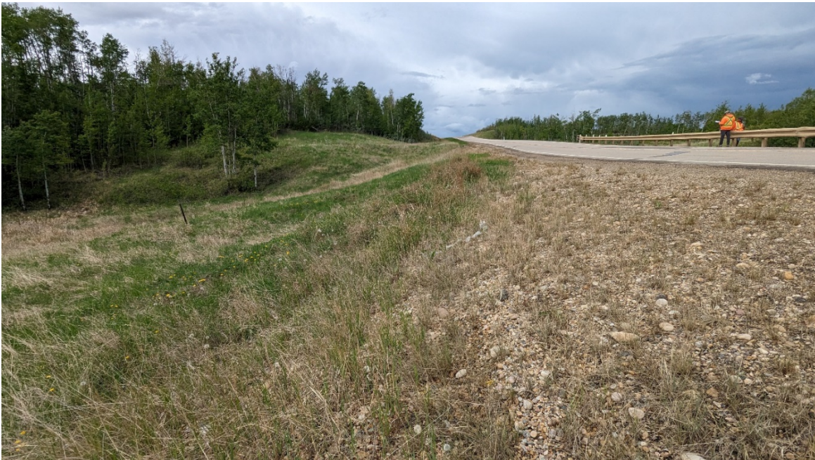
Photo 2 – Looking north at sideslope above culvert inlet.
