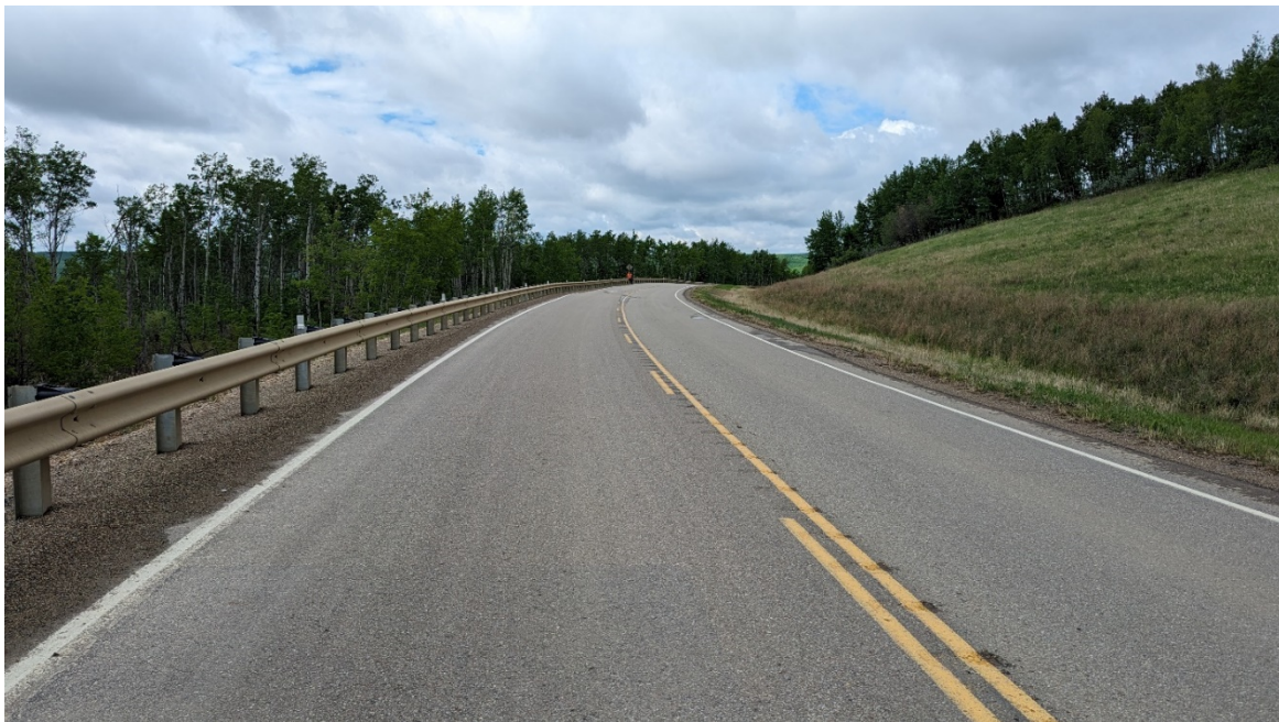
Photo 2, Site 8 – Looking southwest from the northeast end of Site SH012-8. Previous main scarp crack not clearly visible during inspection.
