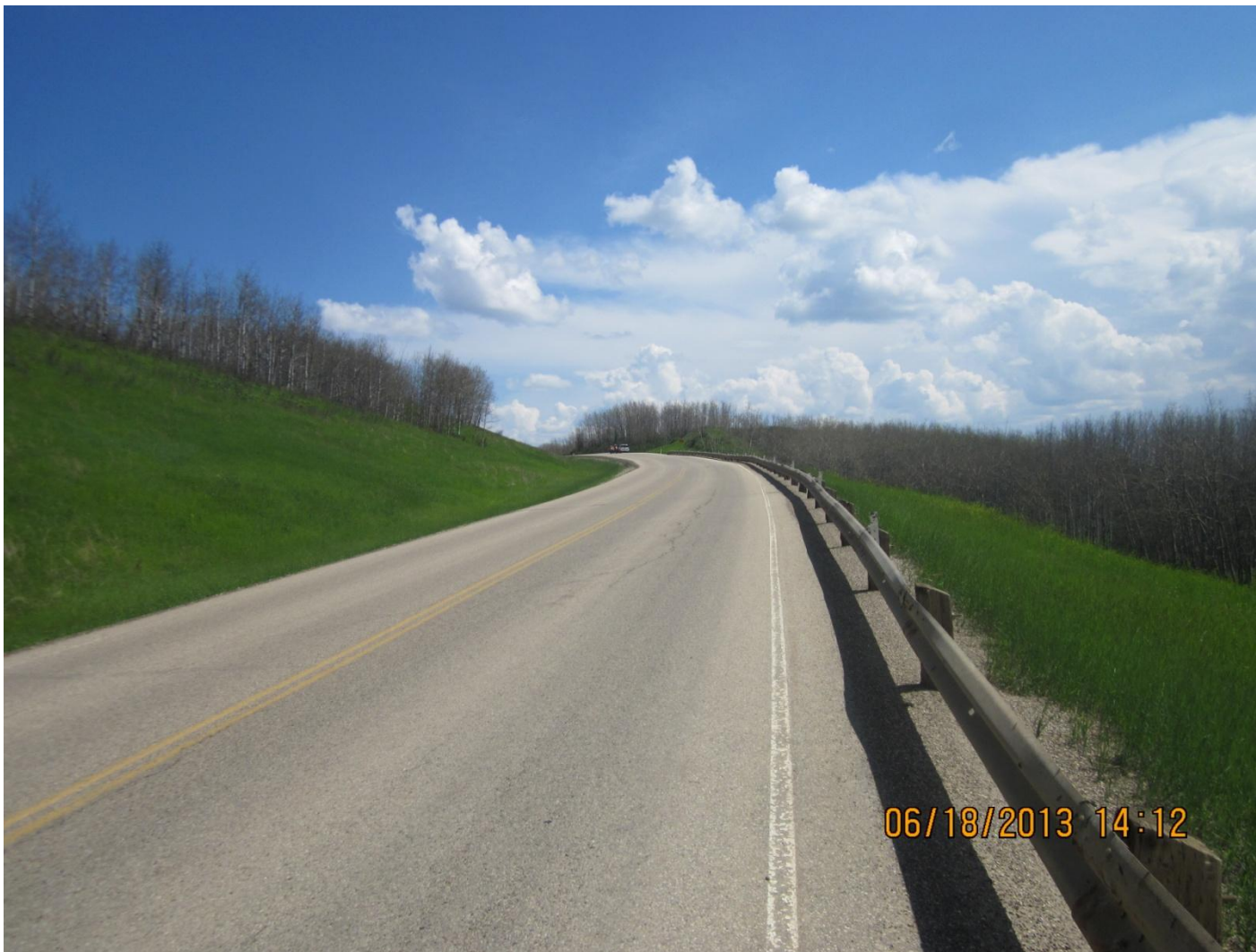
Photo 2: Looking upgrade to the east at the SH11-3 road surface. Note cracking (foreground) and distortion (background).
