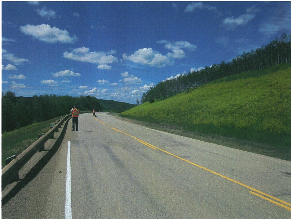
SH11-4 Photo 4. Looking downgrade at SH11-4 (July 2012).
