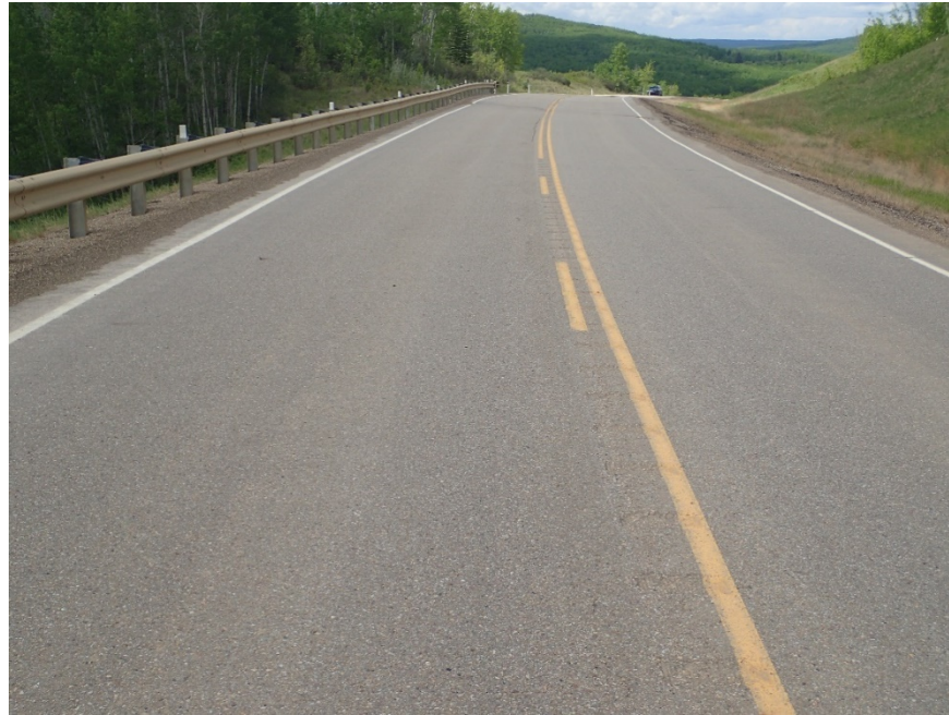
Photo 7, Site 4 – Looking west at ~km 18.82.
