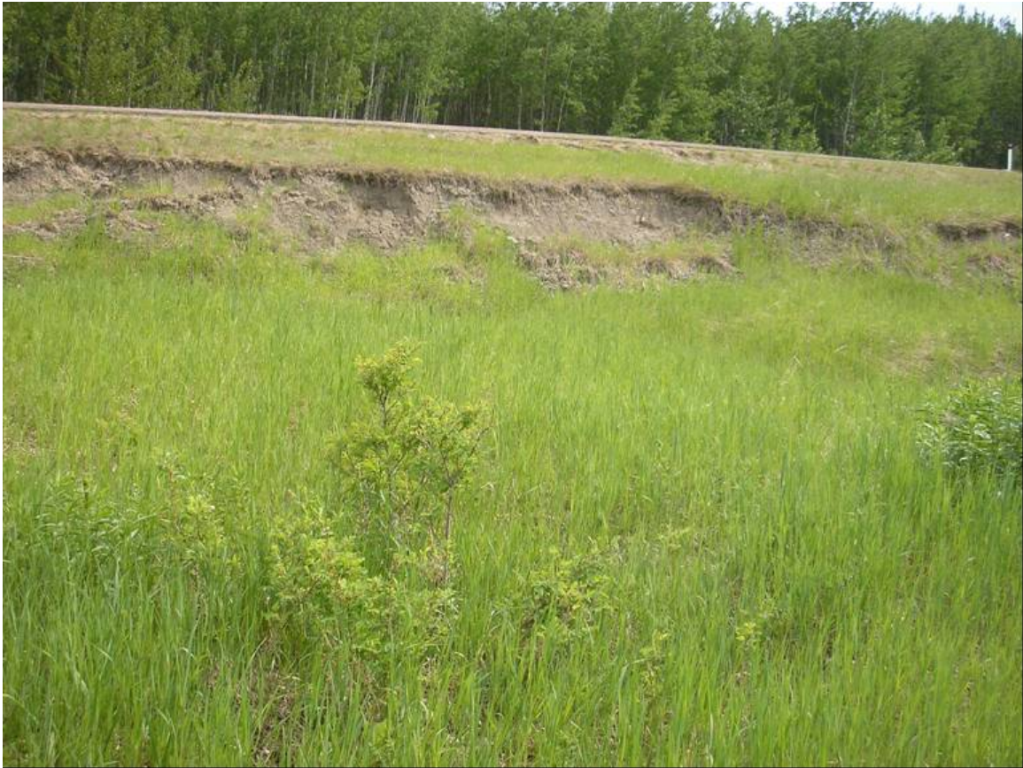
Photo 2 - Looking southeast (upslope) along slide from middle of slump.
