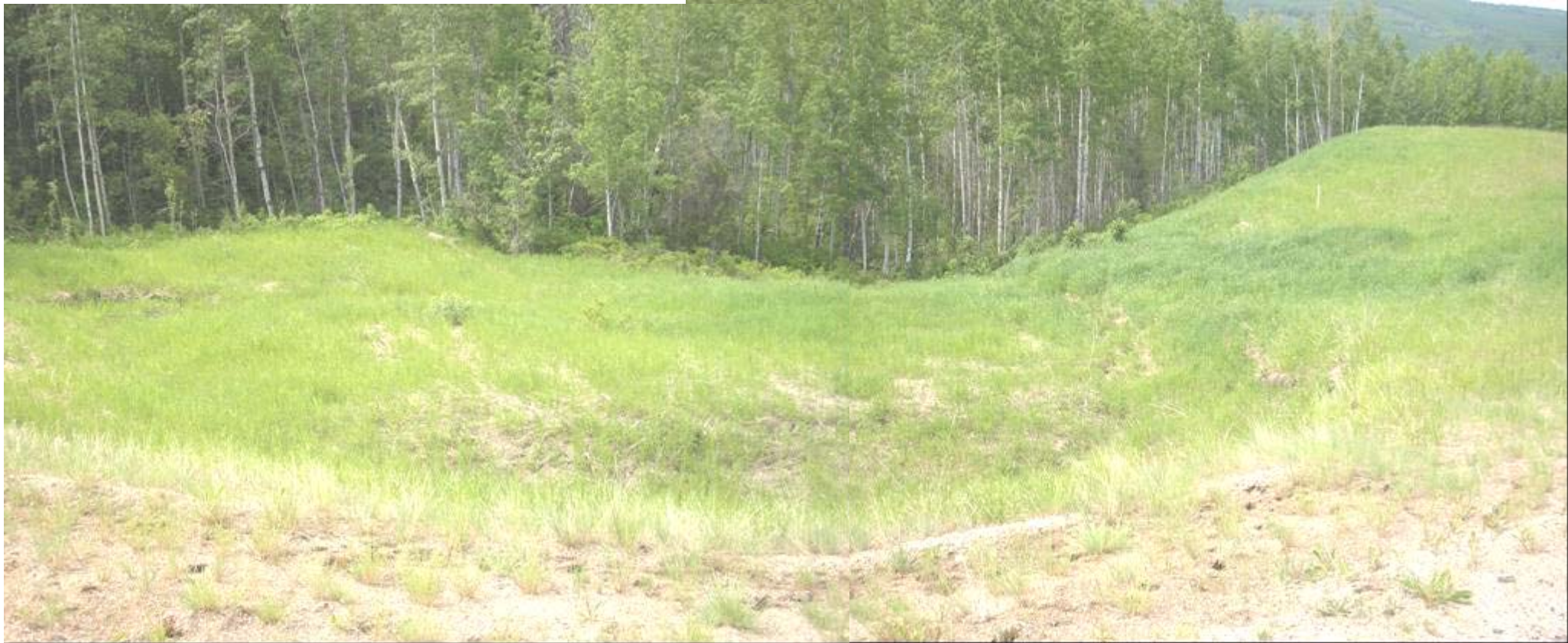
Photo 1 - Looking northwest from south edge of slide, June 14, 2007.
