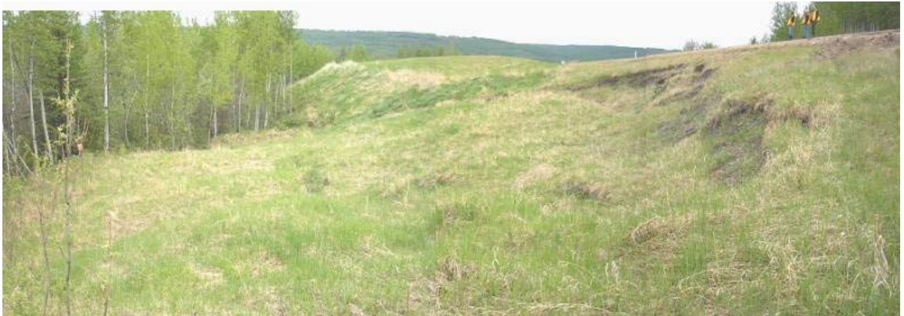
Photo 1 - Looking north from south edge of slide, May 24, 2006.
