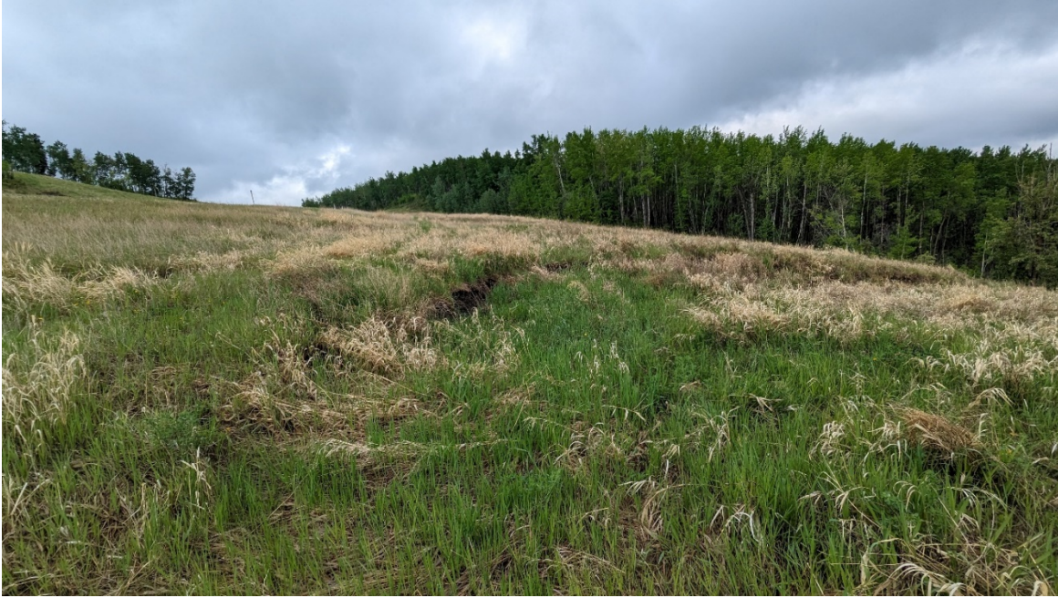
Photo 7 – Looking southeast at scarps downslope of the highway at about km 14.5.
