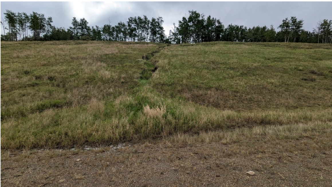
Photo 2 – Looking east at north gully; note slump to left of gully on lower part of slope.
