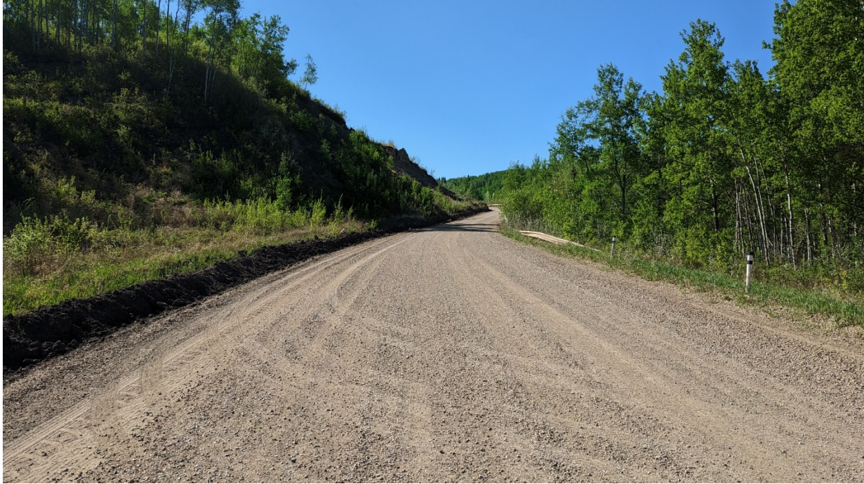
Photo 7 – Looking south towards the south landslide lobe and high shale backslope (PH011-2) on left. The cracks are at the guardrail but had been graded out at the time of the photo.
