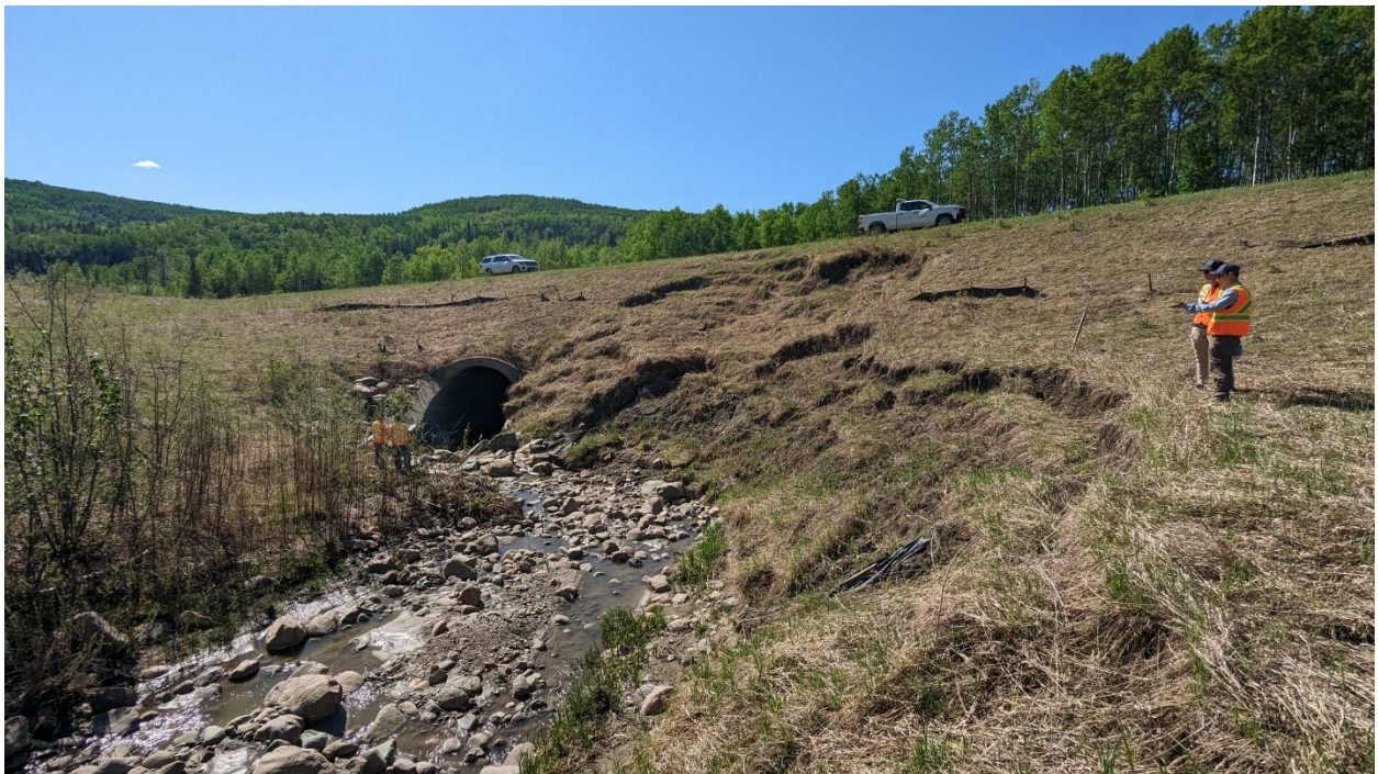
Site 1, Photo 4 – Looking south at culvert inlet.
