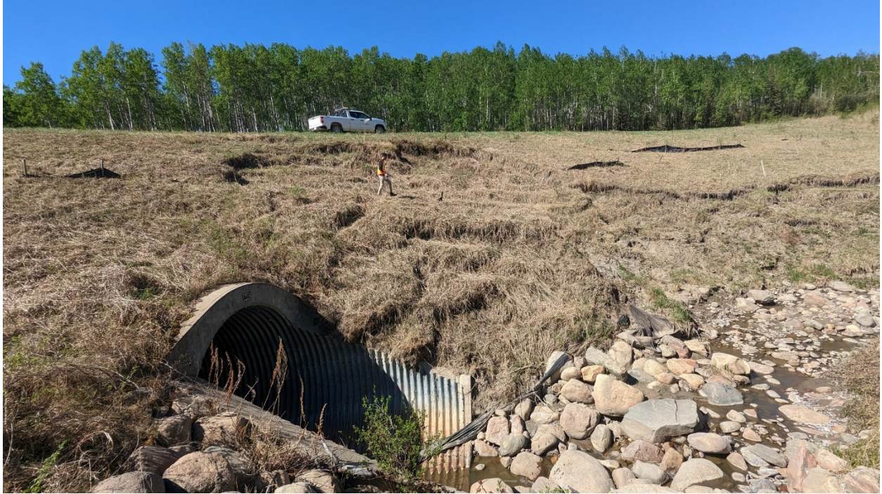
Site 1, Photo 1 – Looking west at north sideslope.
