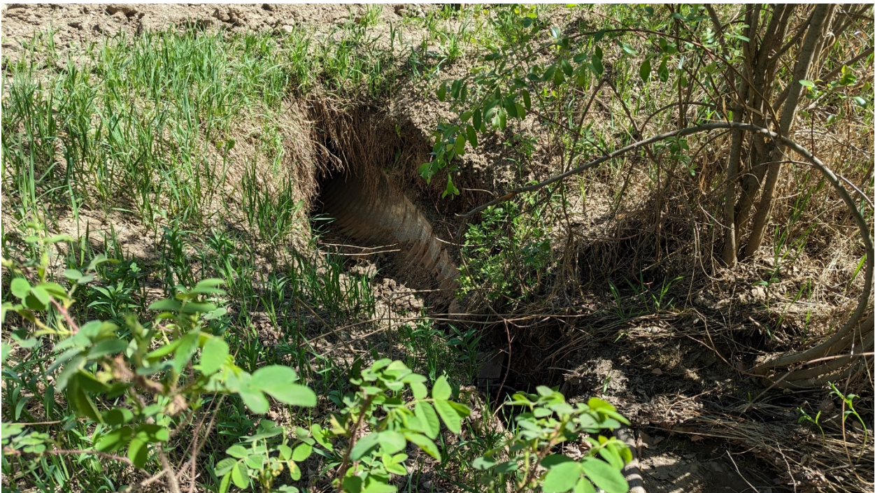
Photo 8 – 900 mm-dia. culvert outlet at the north end of the site.
