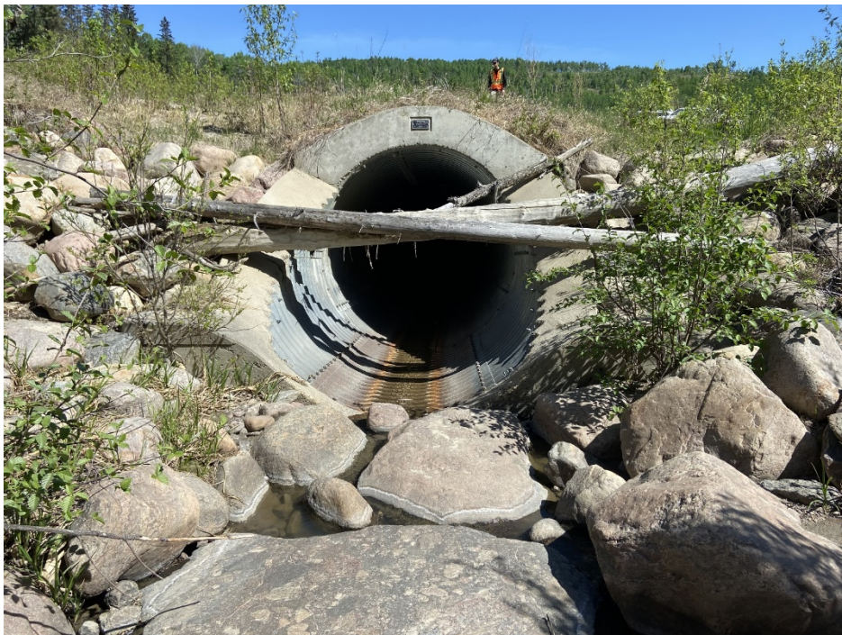
Photo 4 – Looking southeast at culvert inlet.
