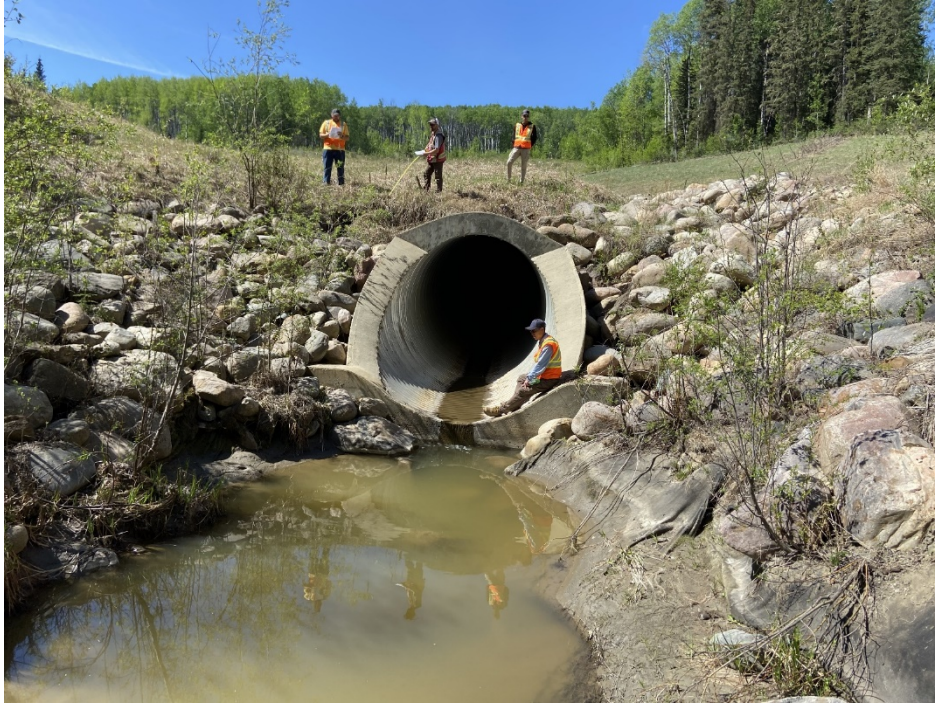
Photo 3 – Looking northwest at culvert outlet.
