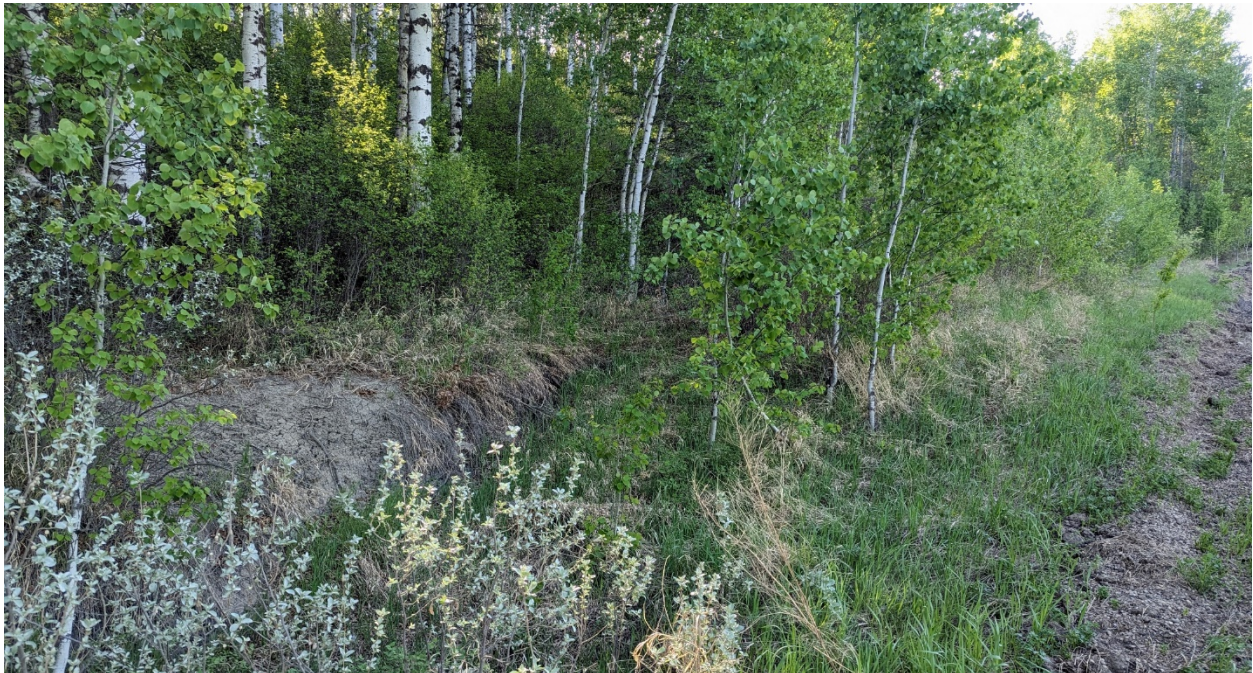
Photo 4 (PH011-3) – Looking south at where displacement has occurred along backscarp of slide at edge of highway.
