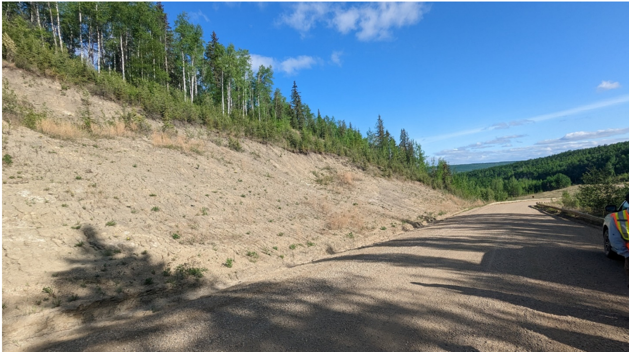
Photo 6 (PH011-1) – Looking at regraded backslope failure area at PH011-1 site (km 42.4).
