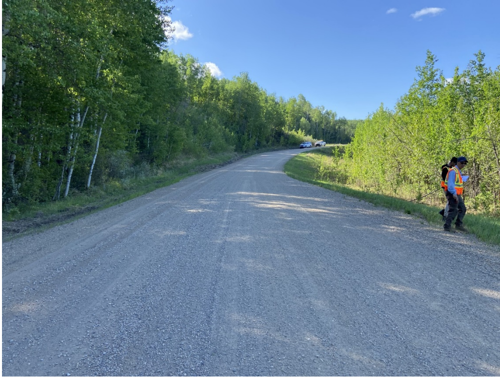
Photo 5 (PH011-3) – Looking south toward the landslide.
