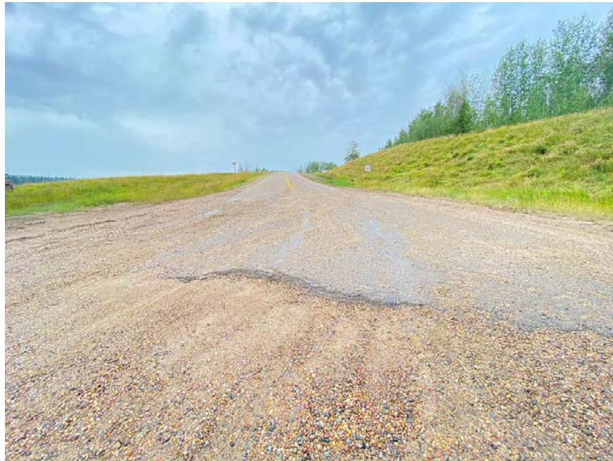
Photo 13. Looking south at end of pavement
