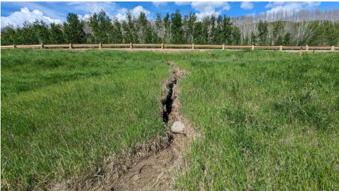
Photo 12 – Erosion gully forming on downslope side of highway at outlet of twin culverts.
