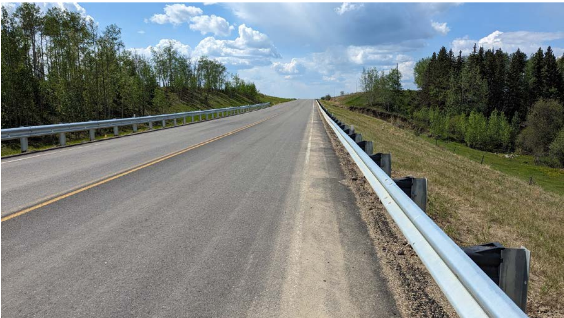
Photo 10 – Similarly, there was no evidence of slumping visible through the recent highway overlay.
