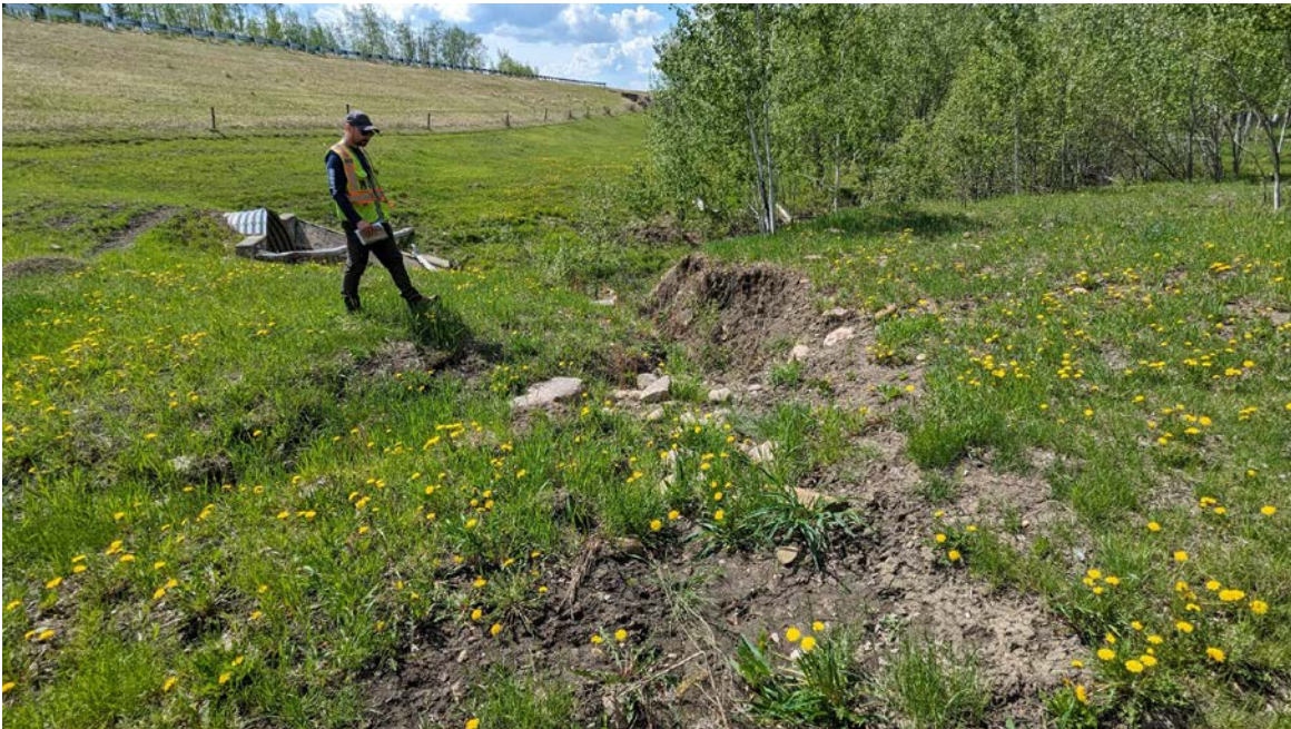
Photo 8 – Looking west at the erosion gully forming near the BF culvert inlet.
