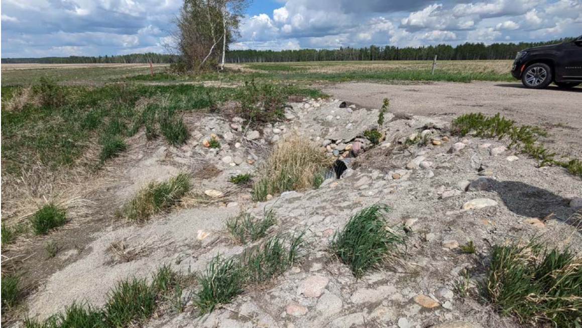
Photo 1 – Grouted riprap at inlet of culvert at km 2.845 approach.
