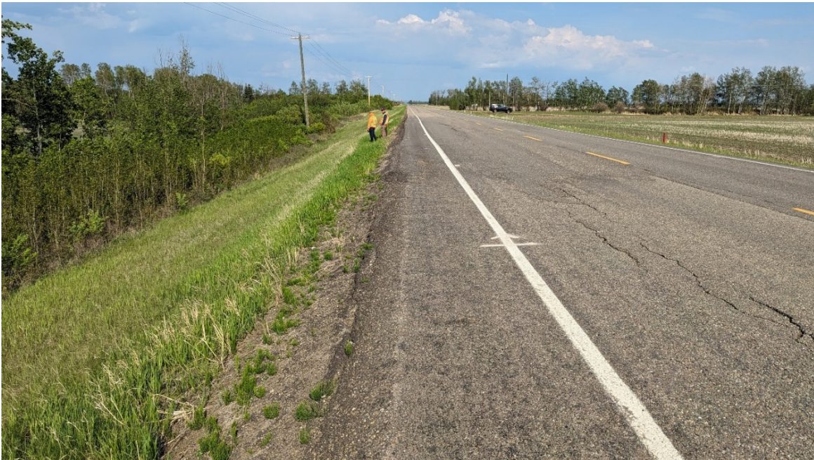
Photo 4 – Looking east from past the previously patched area.
