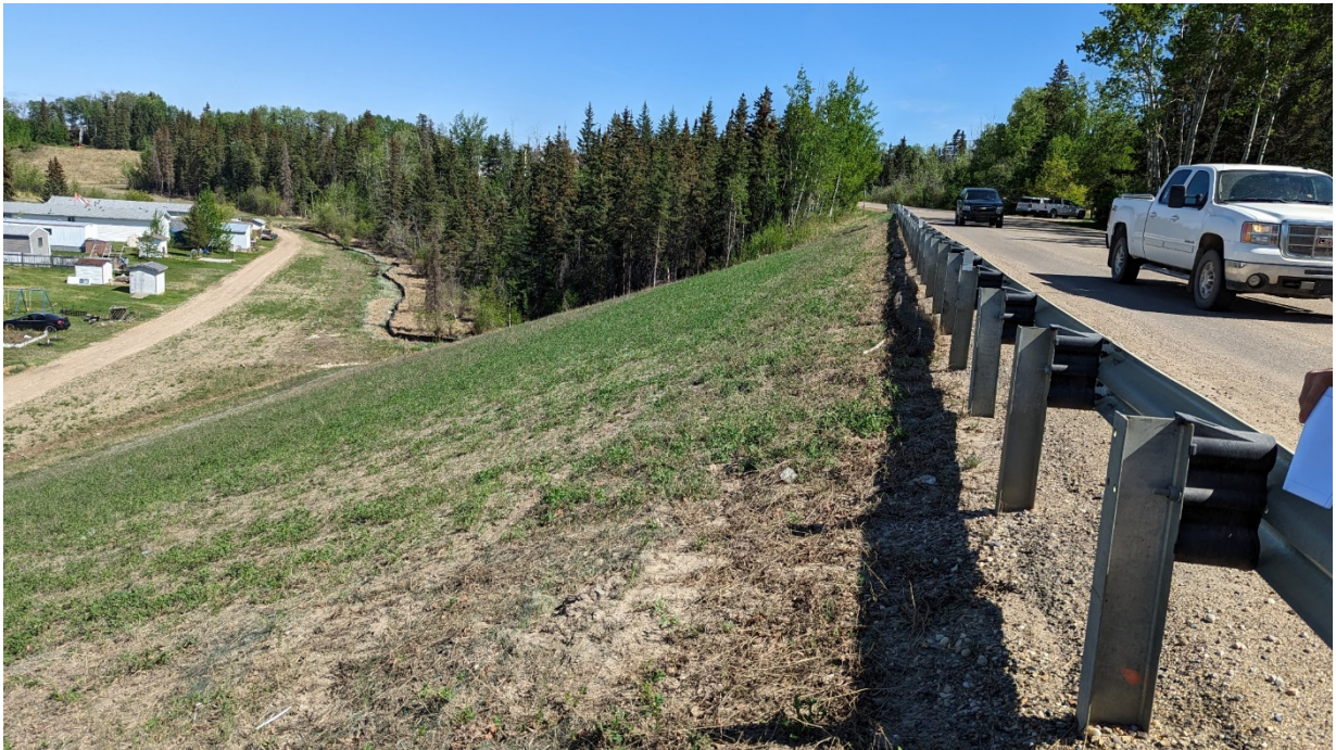
Photo 2 – Looking east along the top of the repaired Hwy 691 slide.
