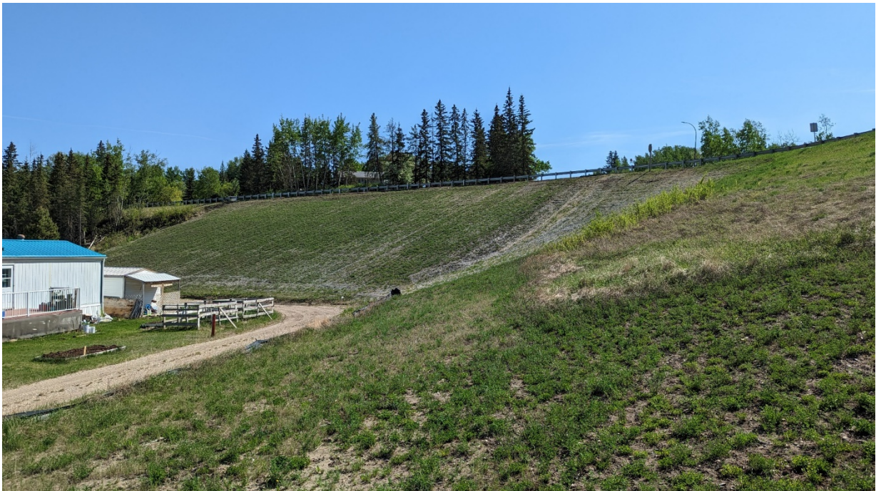
Photo 6 – Looking southeast at the repaired Hwy 691 slide.
