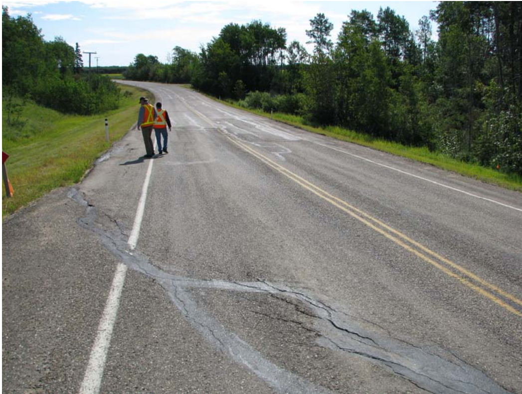
Photo 1 - View of Highway 690 showing the 2008 ACP patch, looking east.
